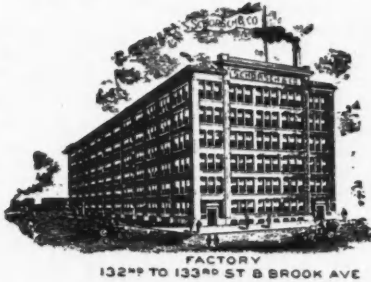
FACTORY 132 ND TO 133 RD ST & BROOK AVE
