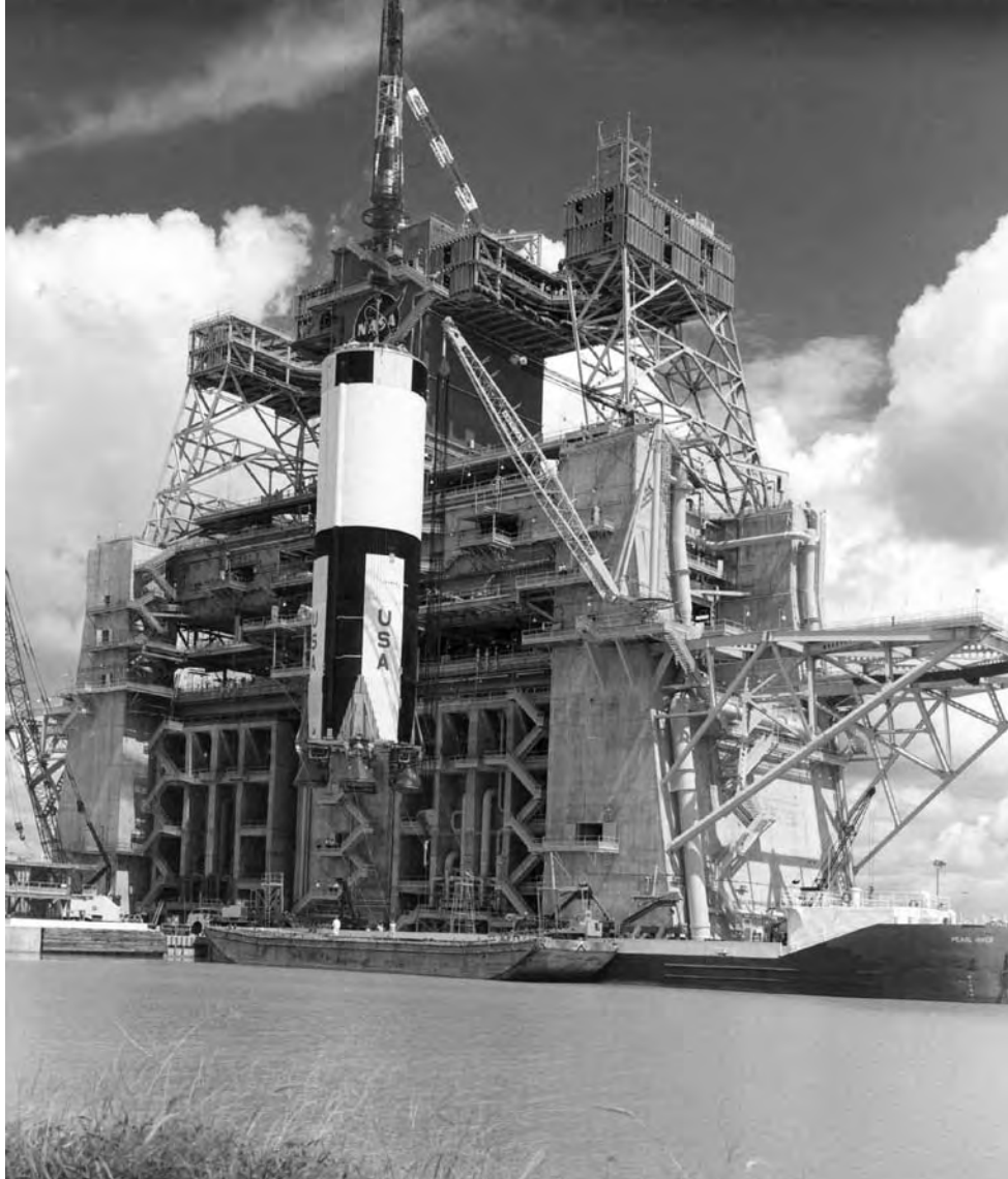
S-1C Stage Installation into Hot Fire Stand at Mississippi Test Facility (MTF) - 1967 (NASA image number: GPN-2000-000559)
