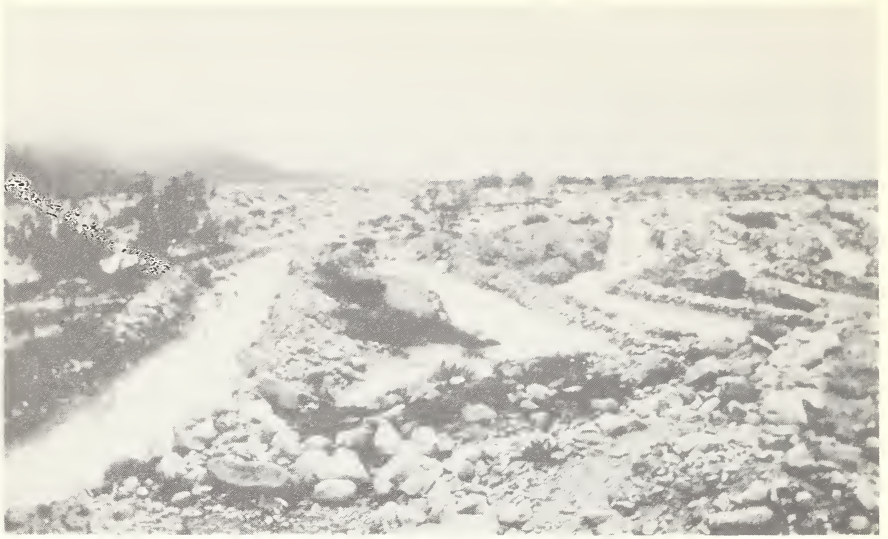
Ditches for recharging purposes. The gravel and boulders increase the infiltration rate.
