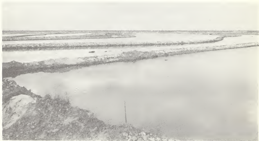
Recharging basins formed by building dikes on the contour.
