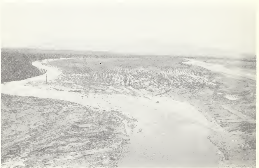
Furrows dug on sandbar of riverbed create a greater wetted area and increase infiltration.
