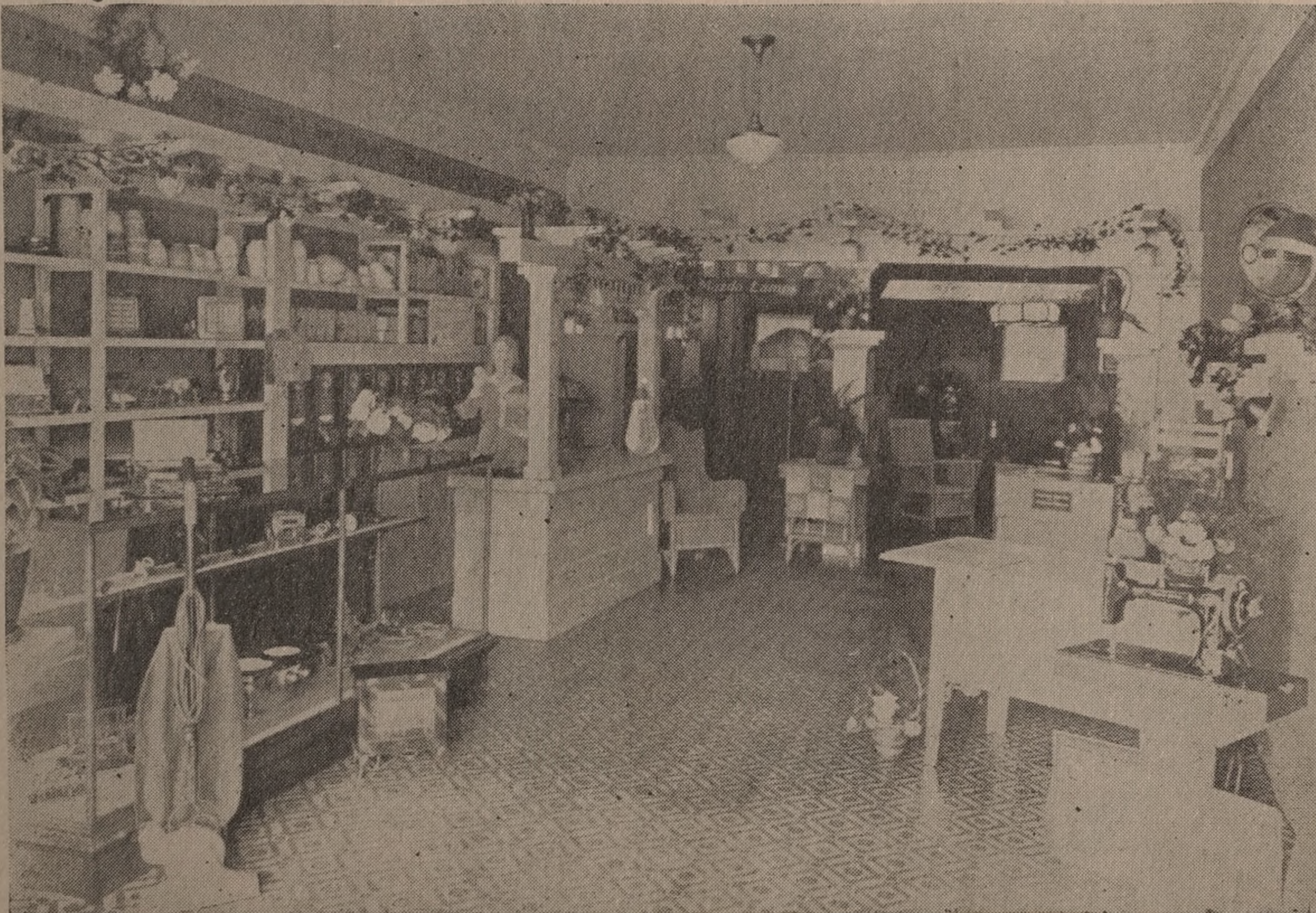
Interior View of Ricker's Live Wire Shop
