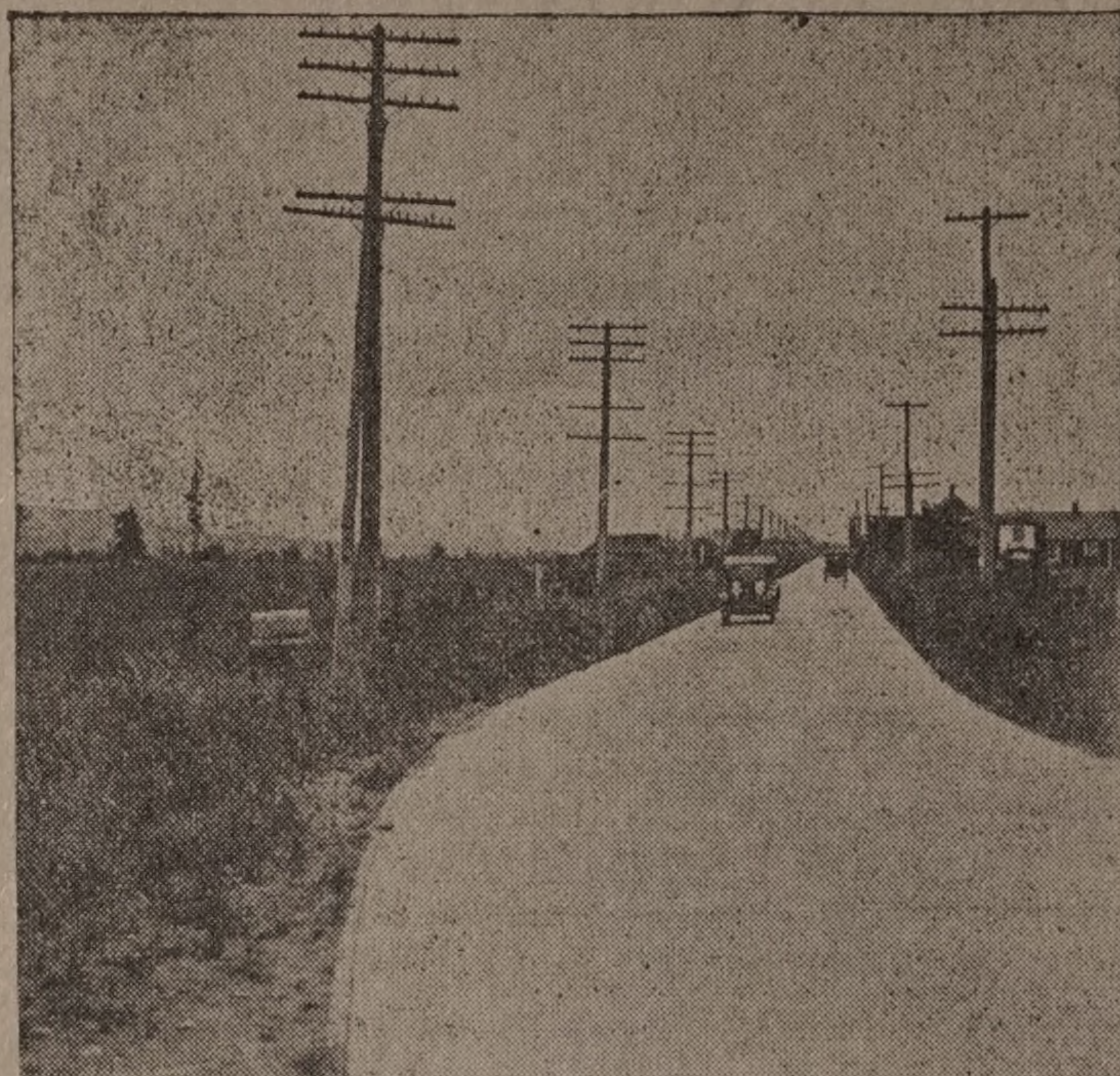
Scene Showing Section of Pacific Highway South of Mount Vernon. Superior Portland Cement Used in Construction
