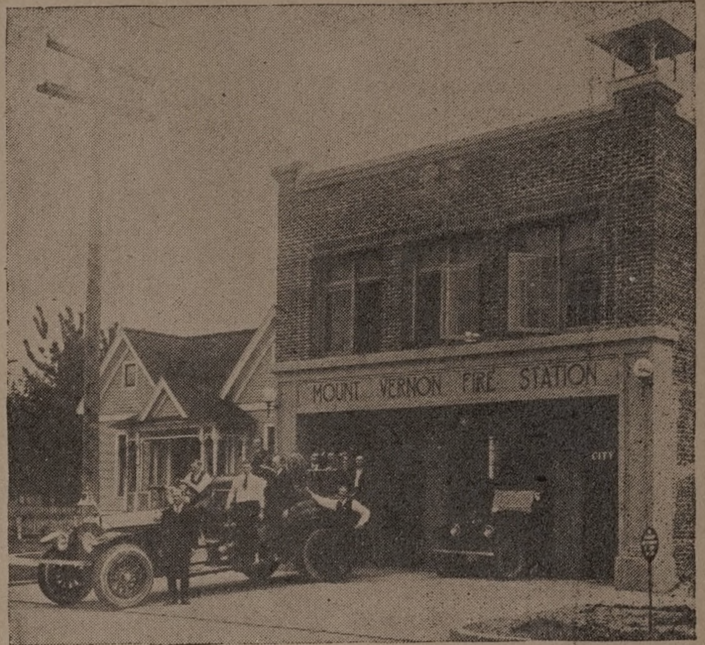
Mount Vernon City Hall and Fire Department
