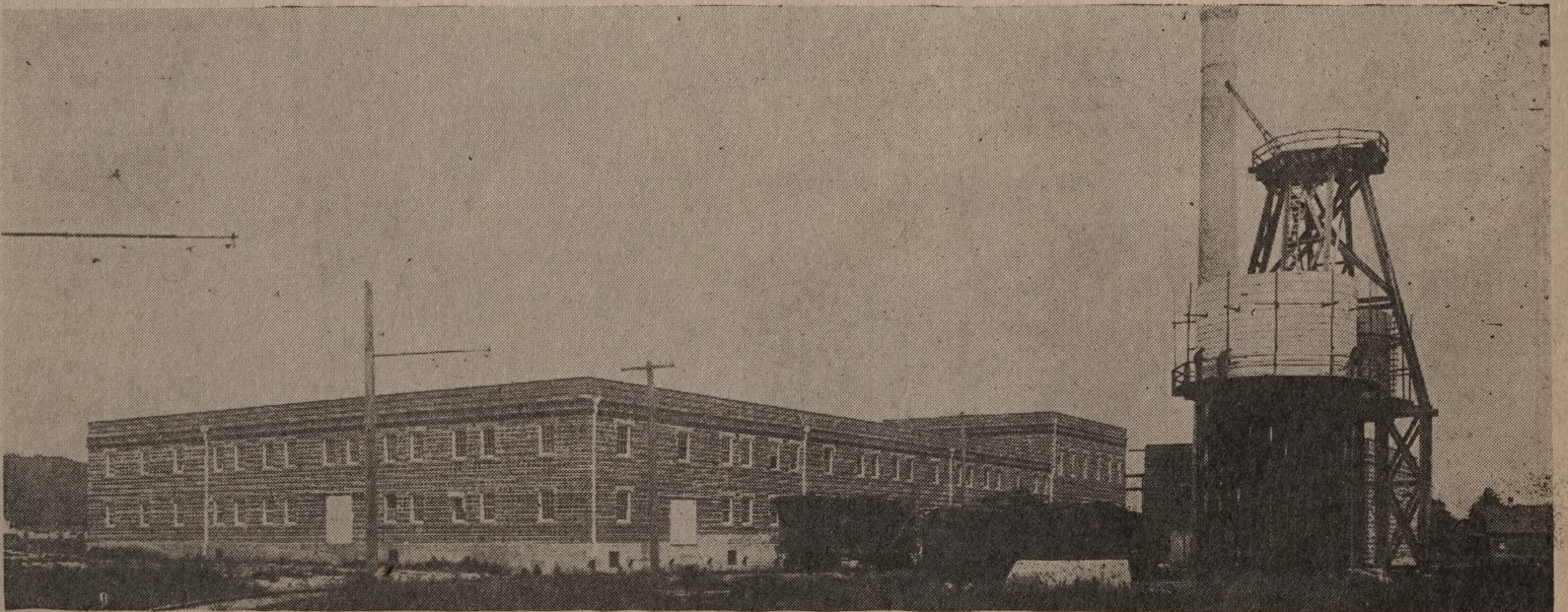
Plant of Skagit County Dairymen's Association, located at Burlington. Grounds comprise seven acres within city limits. Floor space totals 45,000 square feet. Cost when in complete operation will approximate $300,000. T. D. MacNeil, Contractor
