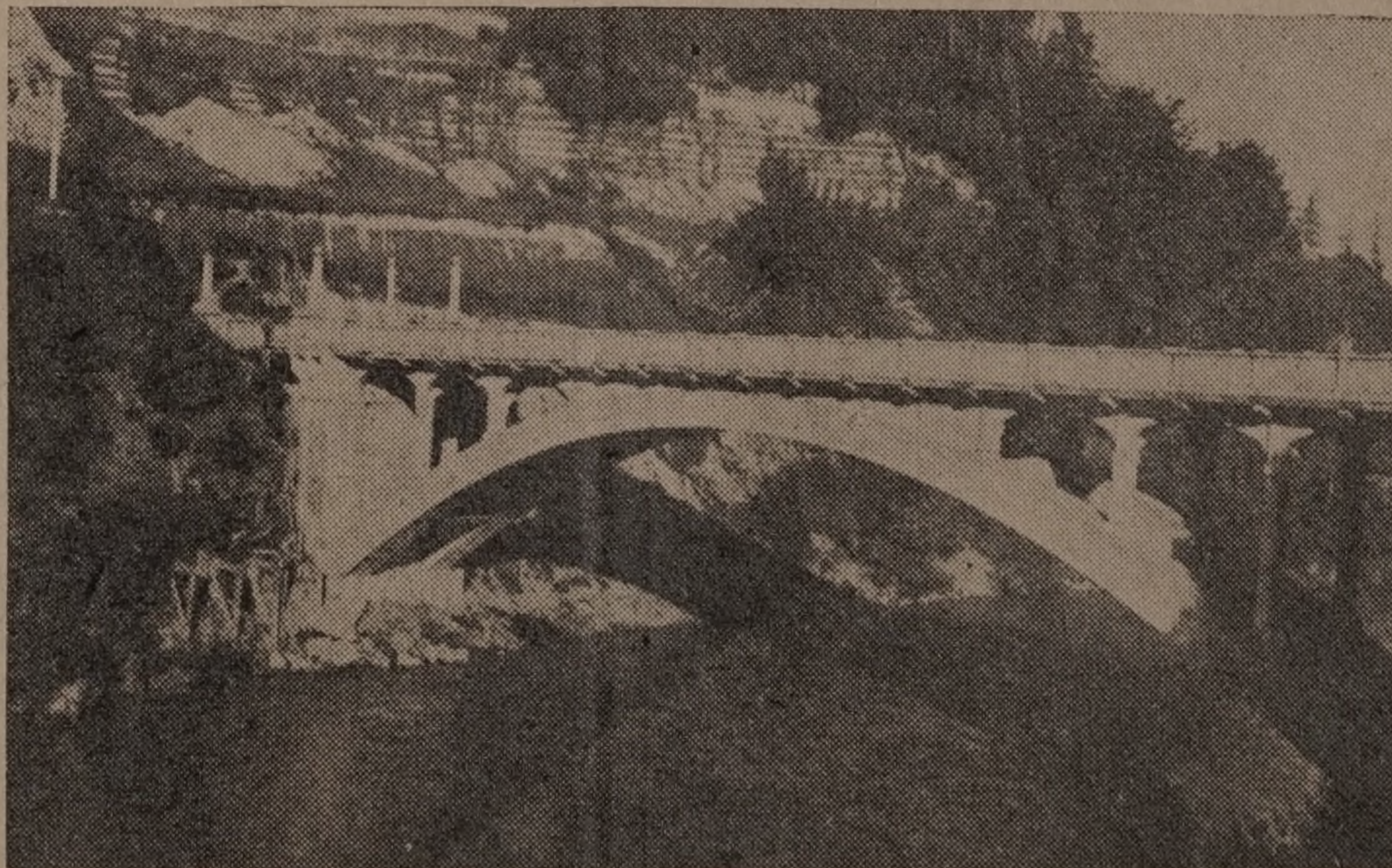
Beautiful Concrete Bridge Over Baker River at Concrete
