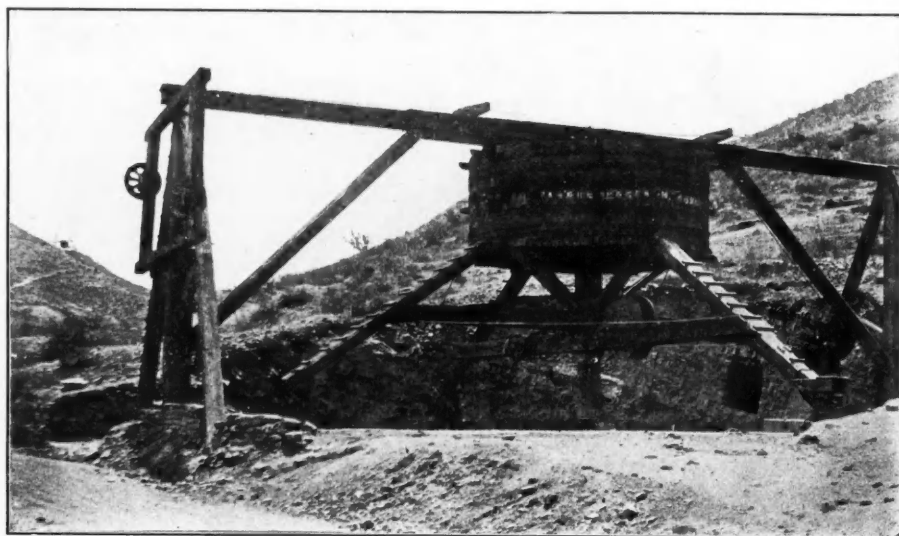
MALACATE, 16 FEET DIAMETER, AT SHAFT 580 FEET DEEP.
