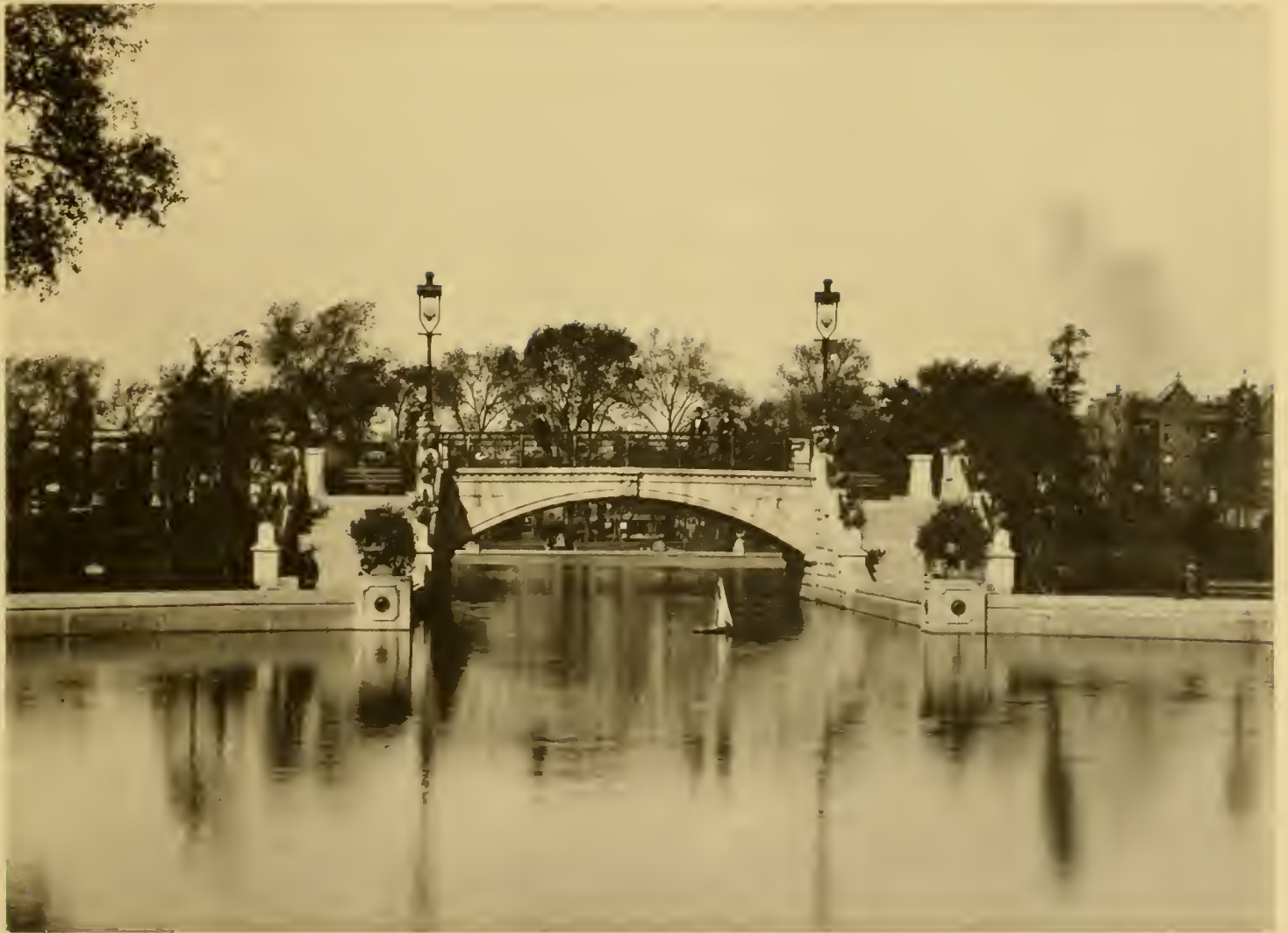
BRIDGE IN UNION PARK.
