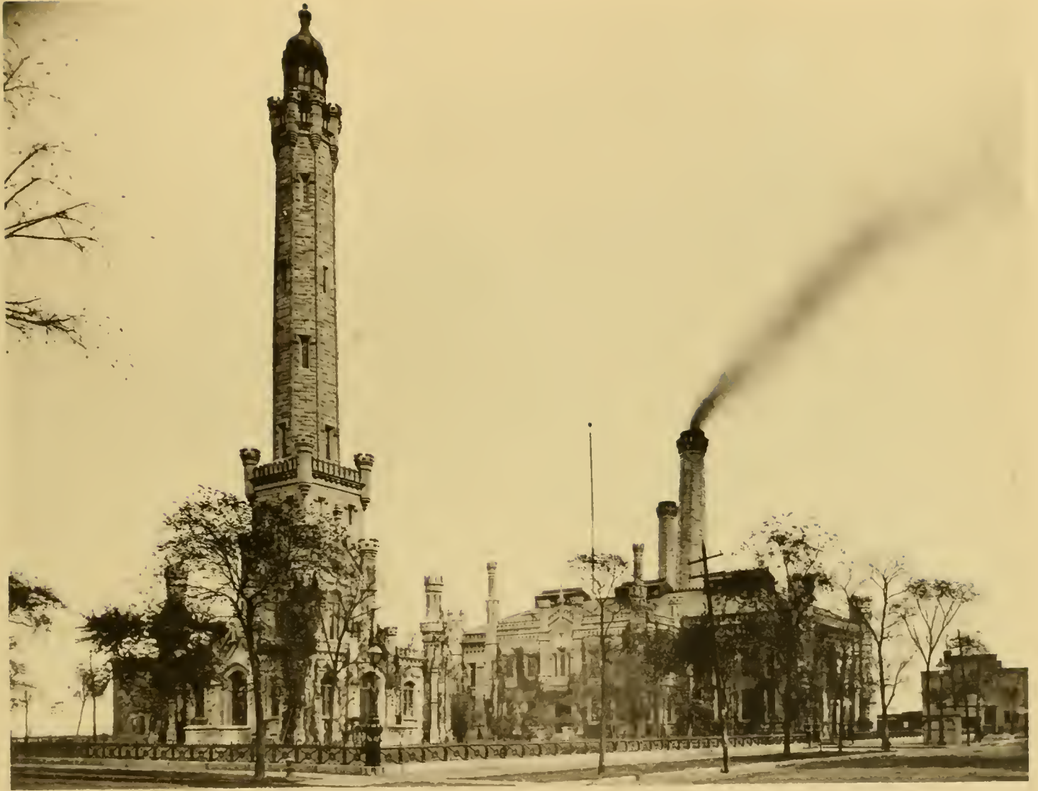
NORTH SIDE WATER WORKS.
