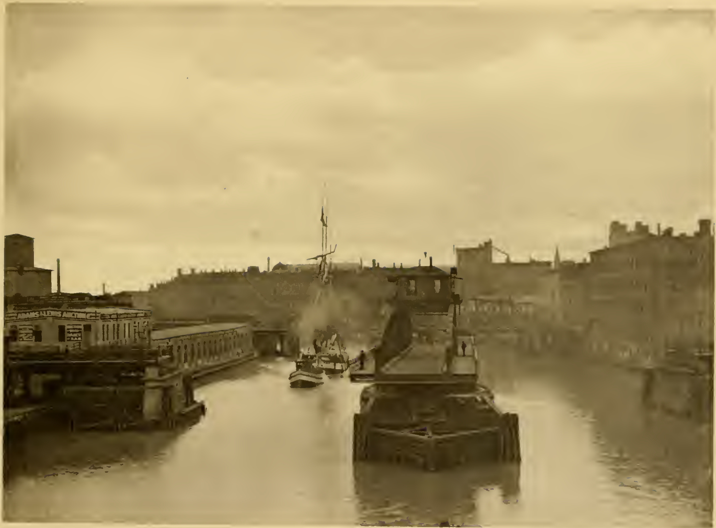
CHICAGO RIVER, from Clark Street Bridge.
