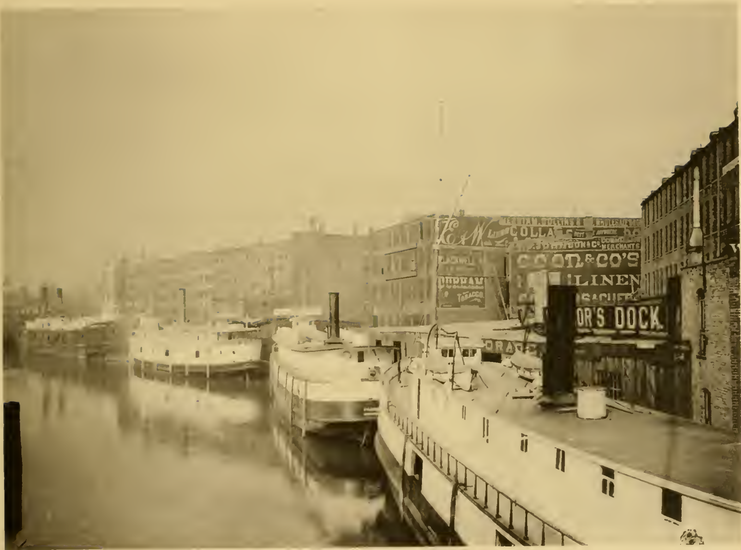
CHICAGO RIVER, East of State Street Bridge.
