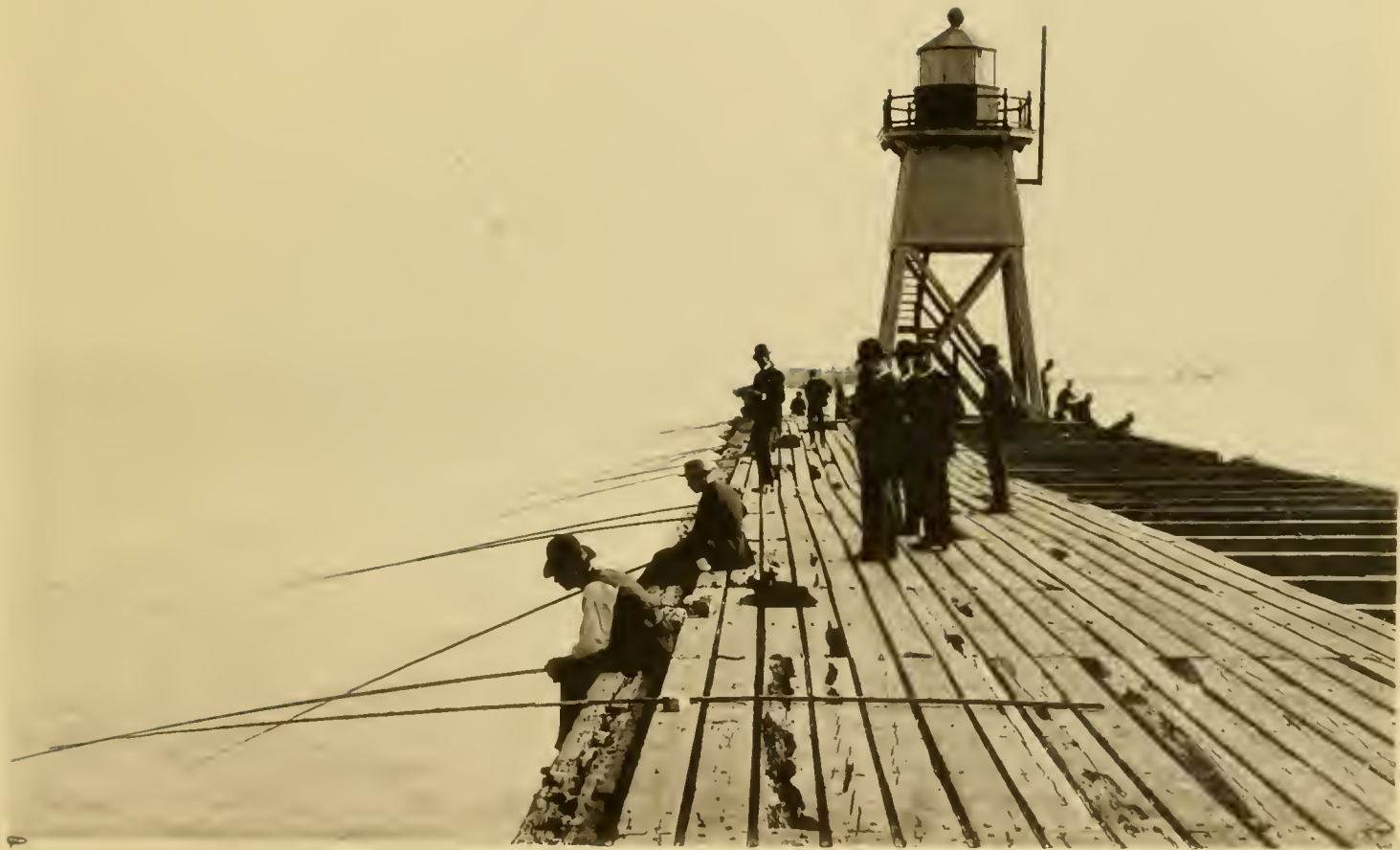
BREAKWATER OPPOSITE LAKE PARK
