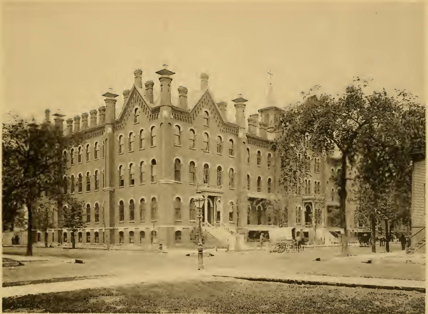
MERCY HOSPITAL, Calumet Avenue and 26th Street.
