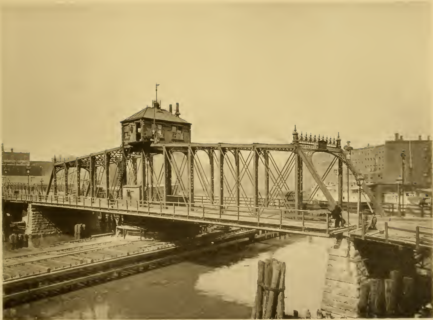
STATE STREET BRIDGE.
