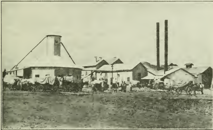
FIG. 35.—Cotton gin in Texas. Each wagon holds enough seed cotton to make a bale of lint weighing about 500 pounds.
