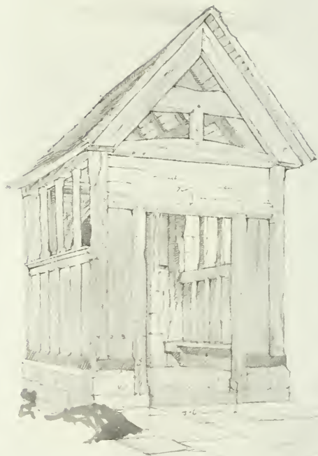
North Porch, Arundel Church, Sussex. A characteristic piece of timber construction.
