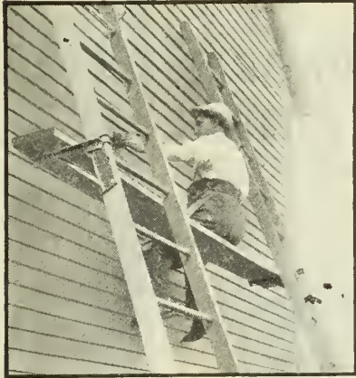
View Showing Jacks on Inside of Ladder
