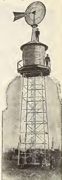
Substructure and Tank with Windmill.
