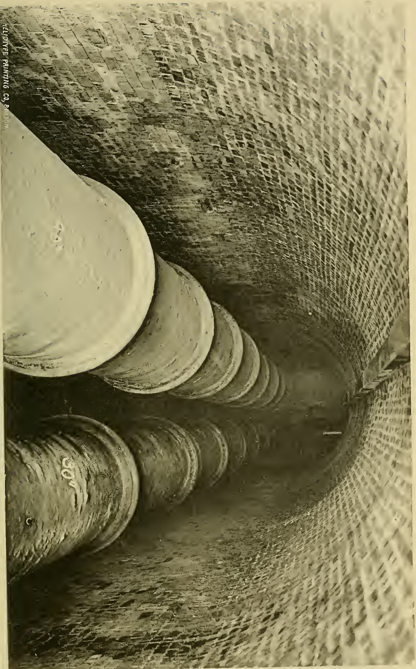
PLATE II. — WATER-PIPE CONDUIT UNDER SECTION 2, BOSTON COMMON, TREMONT- STREET MALL. June 5, 1896.
