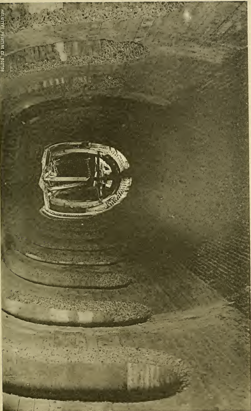
PLATE 28. — UNFINISHED INTERIOR OF SECTION 4, UNDER TREMONT STREET. ONE BARREL OF DOUBLE-BARREL SUBWAY. REFUGE NICHES.
