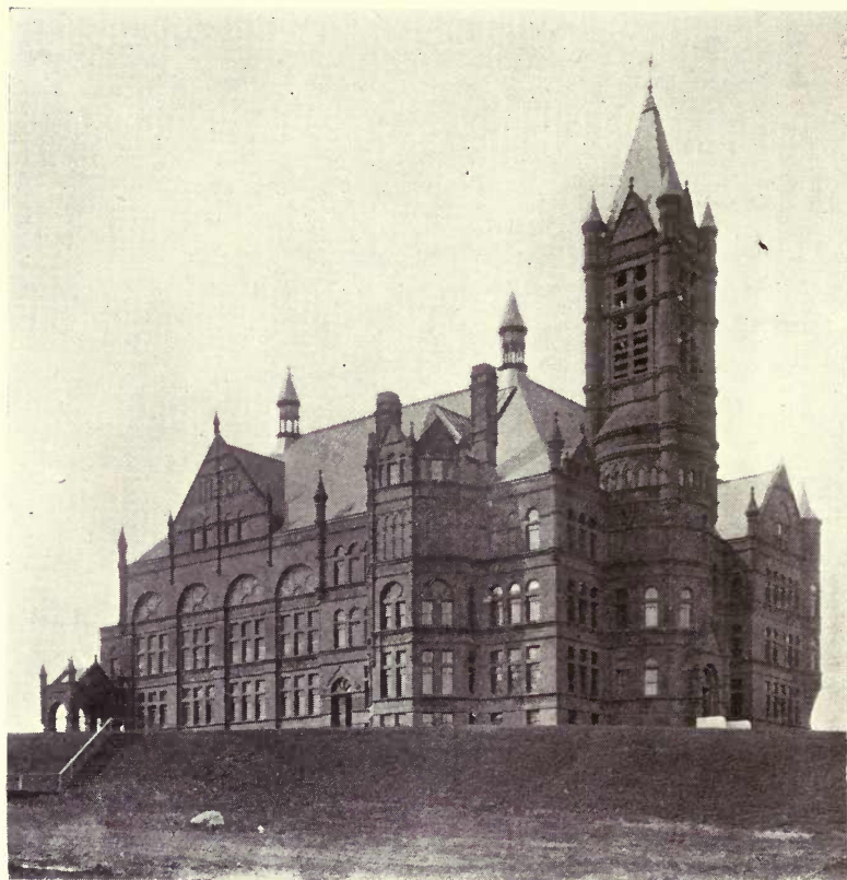
Fig. 219.—Crouse College at Syracuse University, Syracuse, New York, built of Triassic sandstone from East Longmeadow, Massachusetts. Photo. by I. U. Doust.
