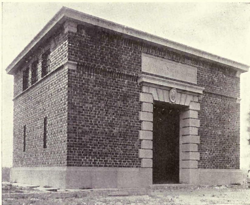
Fig. 306.—Type of building as built for the city of New York by the Board of Water Supply. H. L. Rogers, architect. Catskill aqueduct, portion of the new water system for city of New York. This brick building is trimmed with Onondaga litholite. Photo. furnished by the Onondaga Litholite Company, Syracuse, New York.
