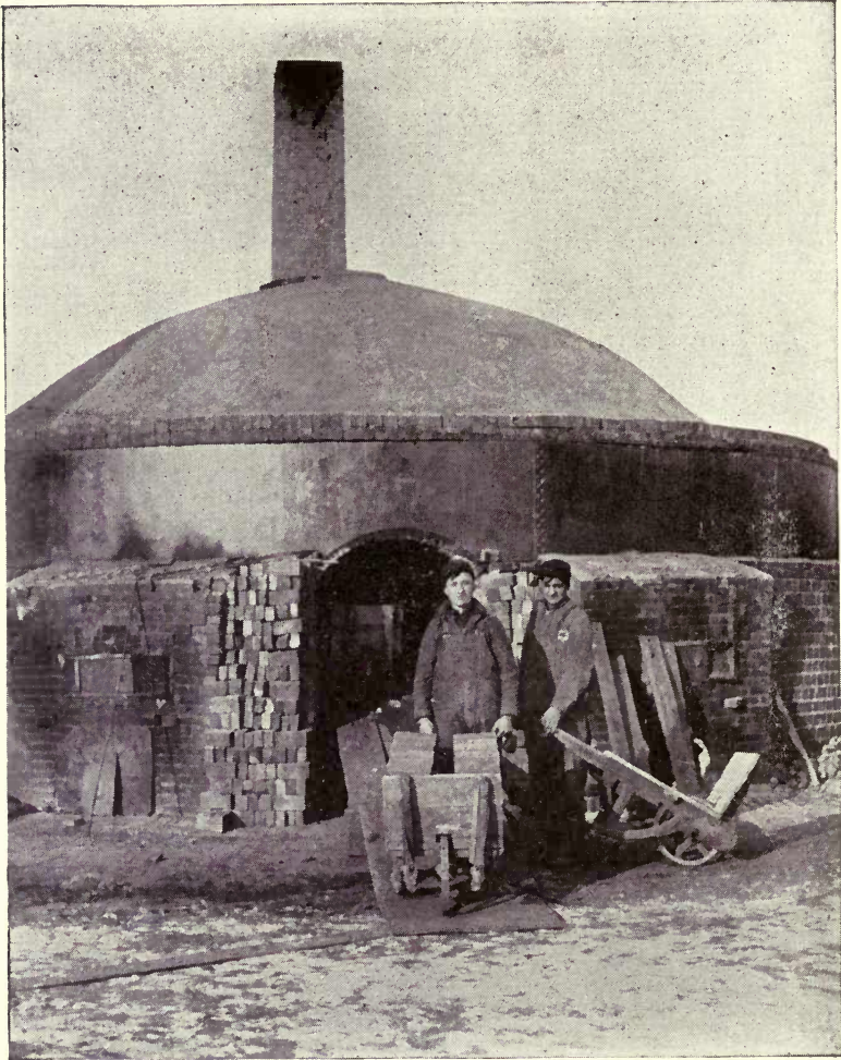
Fig. 293.—Removing the finished brick from a round down draft kiln. By courtesy of the National Paving Brick Manufacturers Association.
