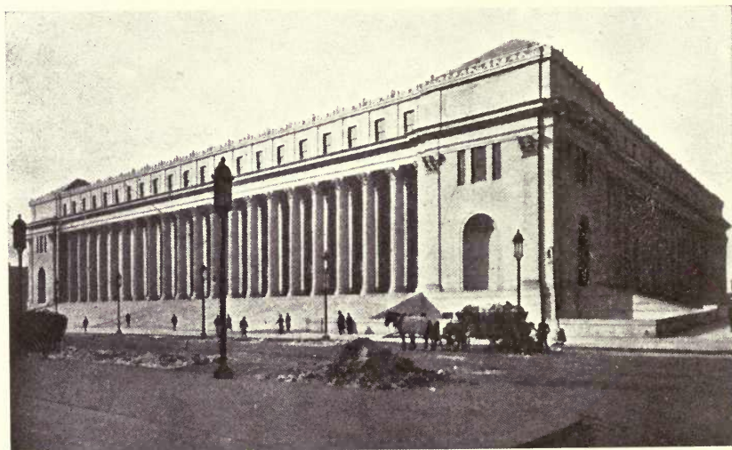
Fig. 45.—United States Post Office, New York City, built of granite from Milford, Massachusetts. By courtesy of the Webb Pink Granite Company, Worcester, Massachusetts.
