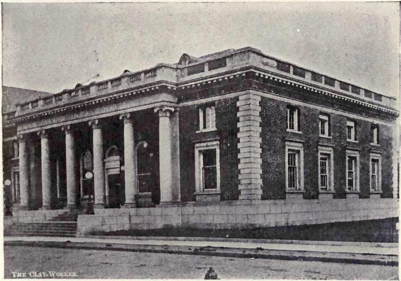
Fig. 273.—Post Office, Bradford, Pennsylvania, built of brick, Oscar Wenderoth, architect. By courtesy of T. A. Randall and Company.
