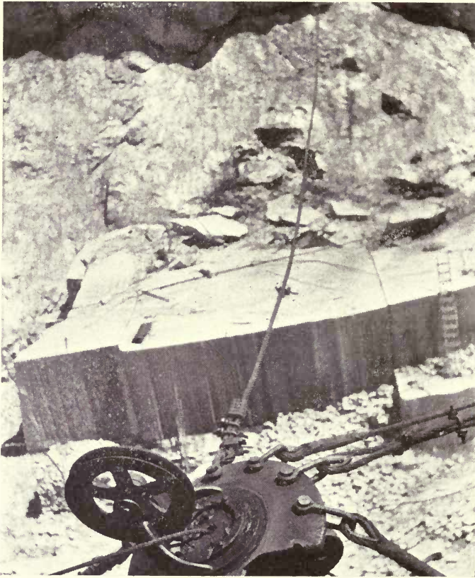
Fig. 73.—A derrick inverted by the removal of the granite too close to a steep wall of mica schist, Barre, Vermont. Photo. by C. H. Richardson.
