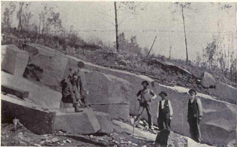
Fig. 65.—Granite quarry, Kirby Mountain, Vermont, showing thickness and dip of sheets. Photo. by C. H. Richardson.
