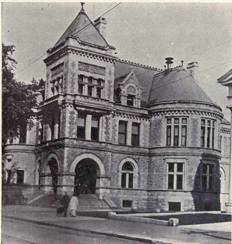
Fig. 208.—Post Office, Montpelier, Vermont, built of Proctor, Vermont, marble. Photo. by C. H. Richardson.
