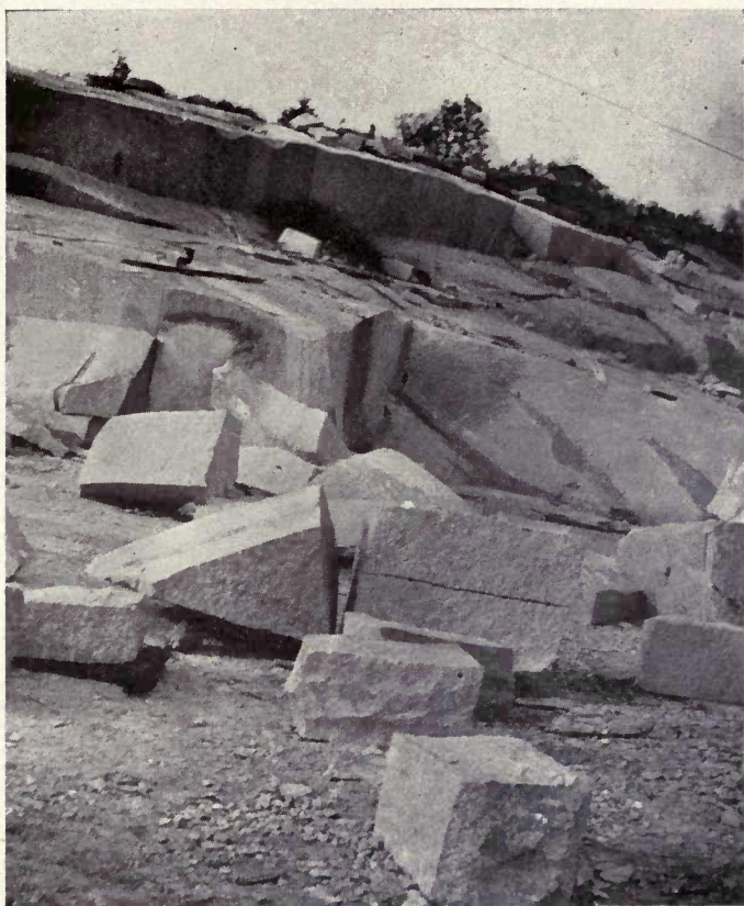
Fig. 85.—Granite quarry of the Woodbury Granite Company, near north end of Robeson Mountain, Woodbury, Vermont, showing thickness and dip of sheets. Photo. by C. H. Richardson.
