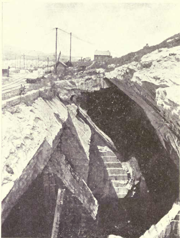
Fig. 160.—View of marble quarry at West Rutland, Vermont, showing dip of the marble beds. Photo. by C. H. Richardson.
