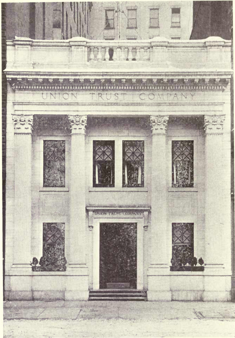
Fig. 99.—Building of Union Trust Company, Rochester, New York, built of Bethel white granite. By courtesy of the Woodbury Granite Company.
