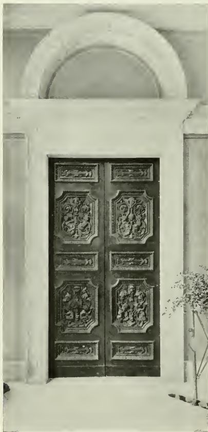
MARBLE DOORWAY IN GALLERY
