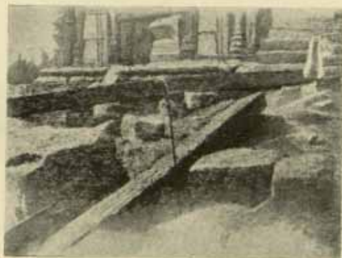
Fig. 1. Iron Beams at Konarak.
