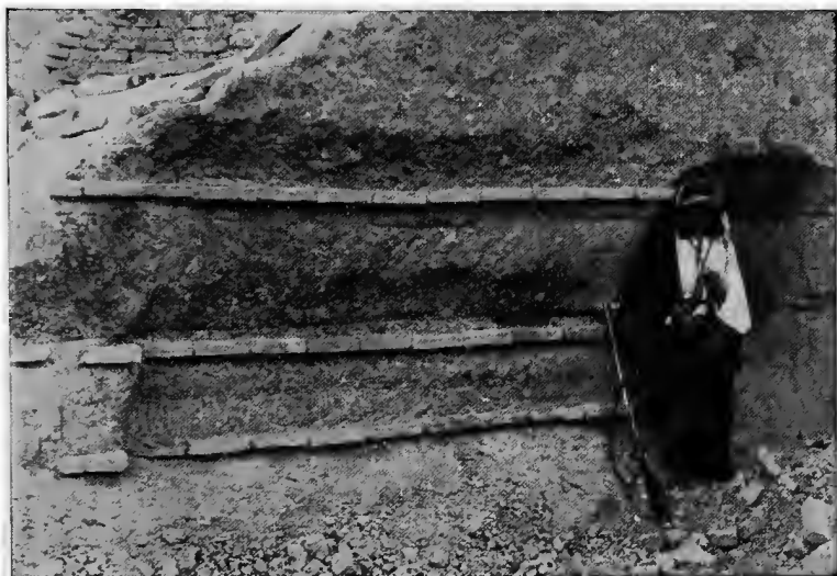
Pavements laid by Ashurbanipal, Kadashman-Turgu and Ur-Niub.
