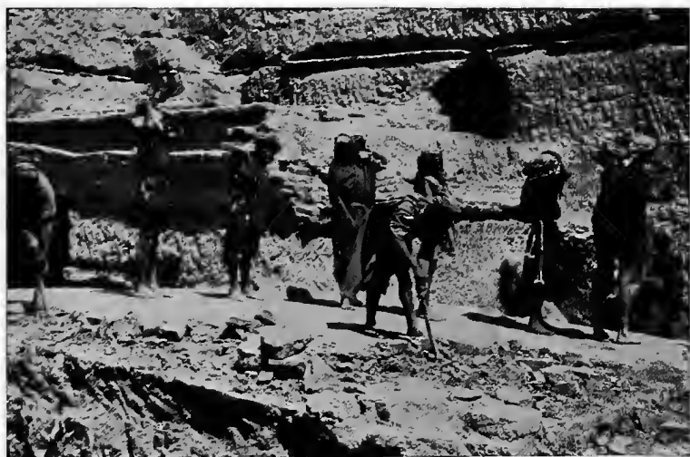
Workman removing the pavement containing bricks with the titles of Sargon and Narâm-Sin.
