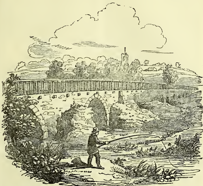
OLNEY BRIDGE, BUCKINGHAMSHIRE.
