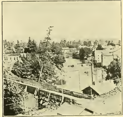
WASHINGTON AVENUE BRIDGE, EAST BRANCH, MAY 1, 1850
