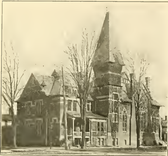
BAPTIST CHURCH CORNER OF MIDDLE AVENUE AND SECOND STREET
