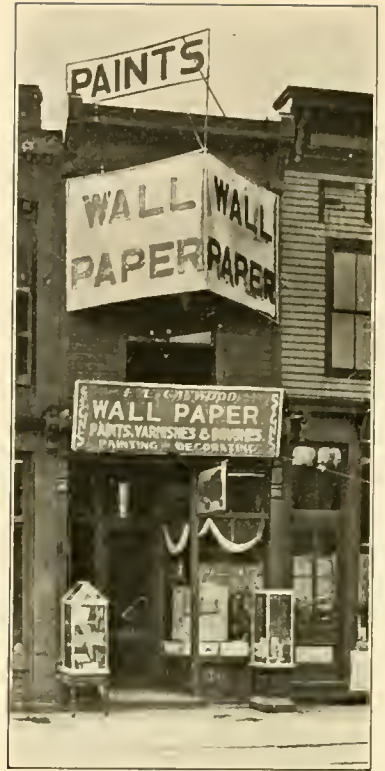
EXTERIOR VIEW OF CAYWOOD'S STORE
