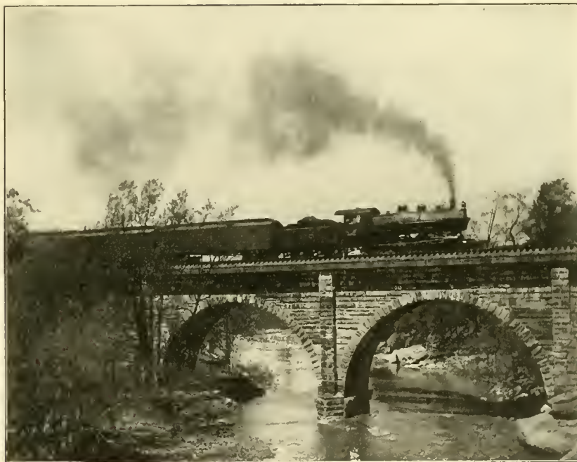
RAILROAD BRIDGE OVER EAST BRANCH OF BLACK RIVER
