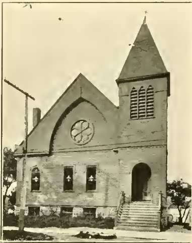
SECOND CONGREGATIONAL CHURCH CORNER OF LODI STREET AND LAKE AVENUE
