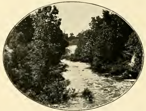
VIEW OF WEST FALLS FROM CABLE BRIDGE
