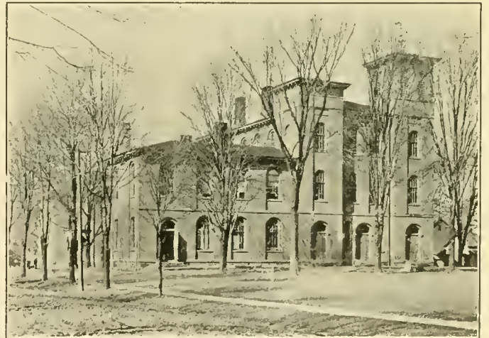
RIDGE STREET BUILDING
