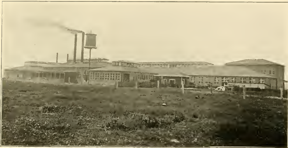
The above picture is a view of the new Columbia Steel Works, built by F. E. Wolf, contractor. Mr. Wolf has built many of the substantial blocks and residences of Elyria.
