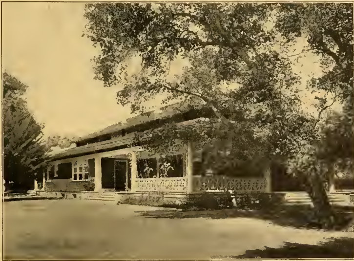
Clubhouse Paso Robles Hot Springs Hotel.
