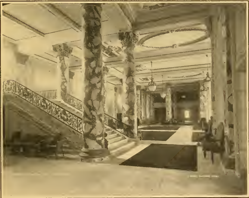
The Marble Lobby of the Fairmont excels all others in height and spaciousness.
