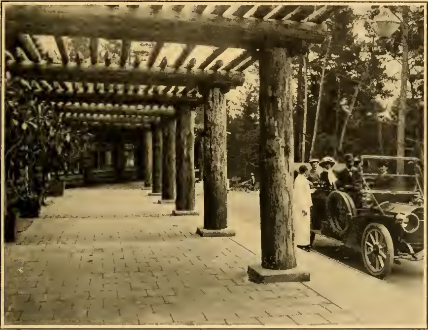
Pergola and Porch of Pebble Beach Lodge Note the massive log pillars.
