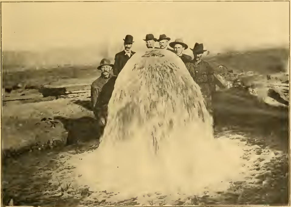
The City's Artesian Well, San Bernardino, Cal. This well flows three million gallons every 24 hours.
