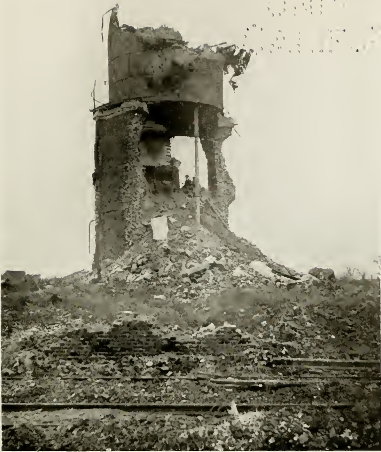
WATER TOWER O.P., VERMELLES.
