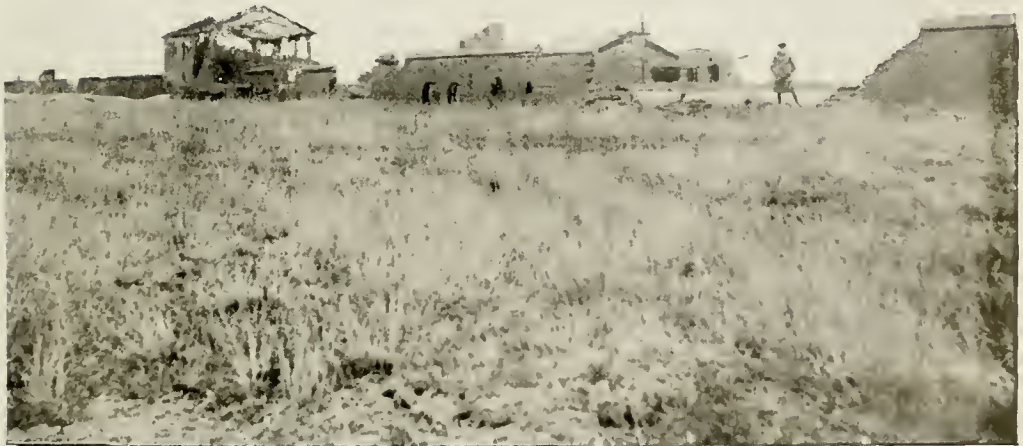
BATTERY POSITION AT VERMELLES.
