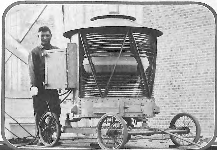
Half-billion candle-power flood-light used to illuminate landing fields. (Below) How the fields look lighted up
