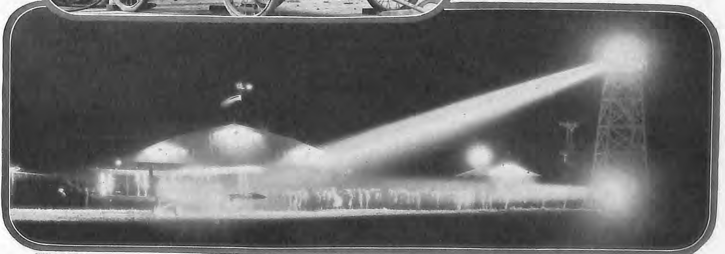
Half-billion candle-power flood-light used to illuminate landing fields. (Below) How the fields look lighted up
