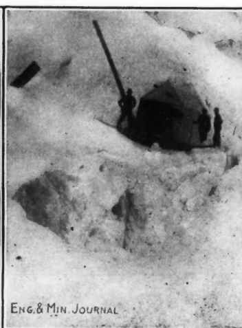
ON SHOUP'S GLACIER Taking donkey engine around crevasse with blocks and cable.
