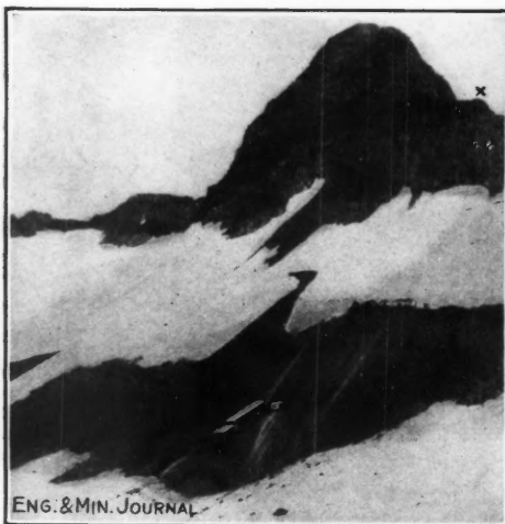
UPPER VEIN, GOLD KING MINE Ore is let down from point (X) to mill, over snow in sleighs.
