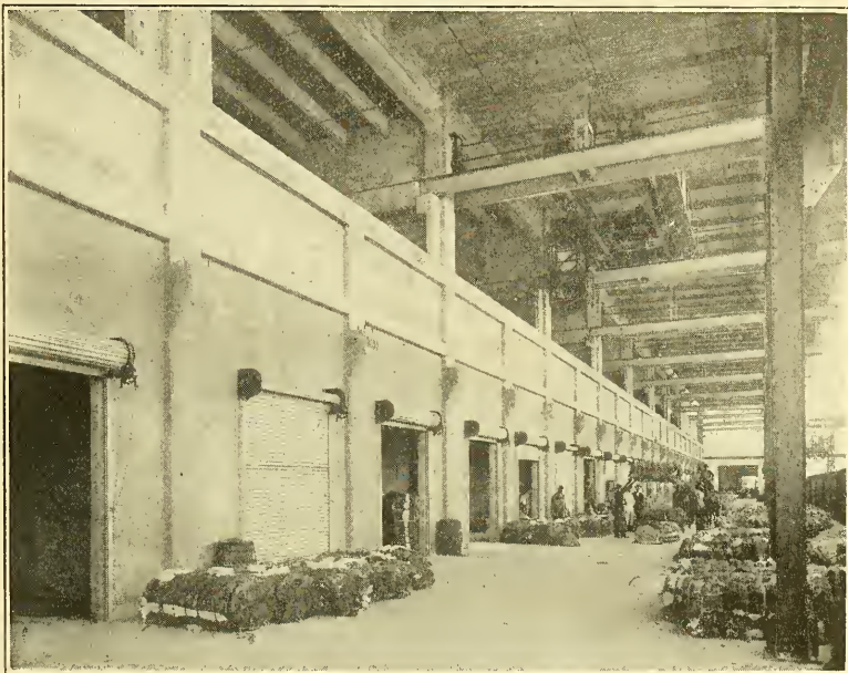
Interior View of Cotton Warehouse.
