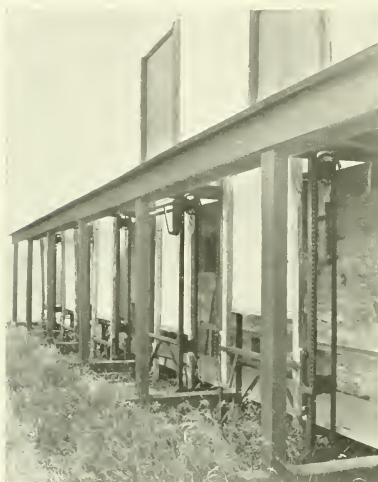
BEHIND THE RIFLE BUTTS, SHOWING MECHANISM OF THE TARGET-LIFTS
