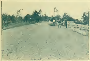
A portion of the Long Island Motor Parkway under construction
