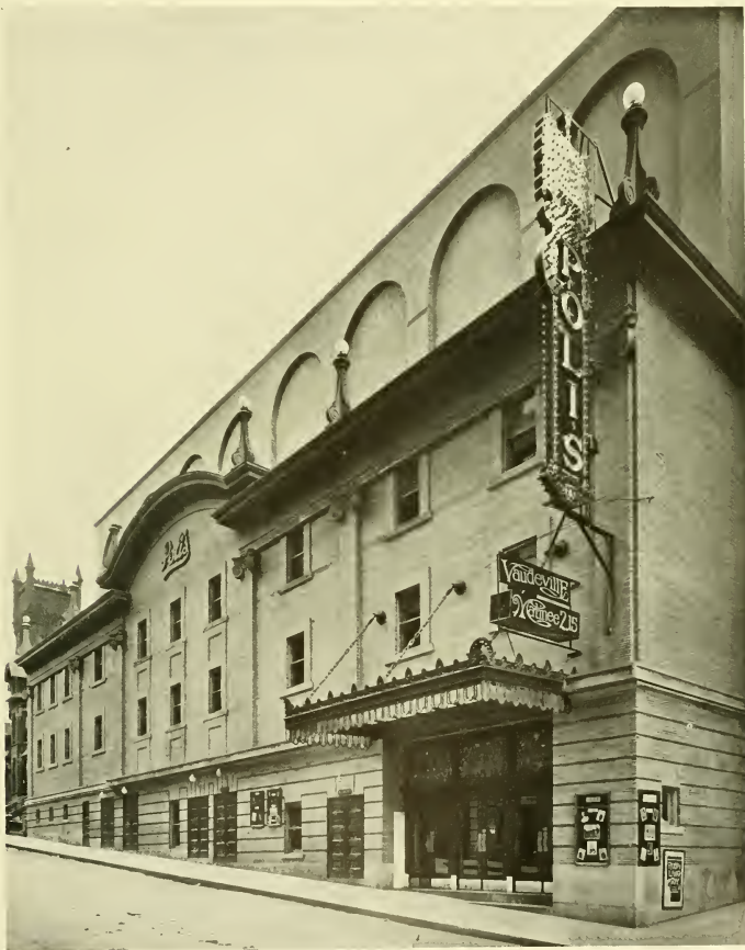
EXTERIOR OF NEW POLI THEATRE ON ELM STREET
