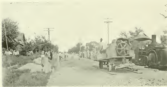
HASSAM PAVEMENT IN PROCESS OF CONSTRUCTION.
