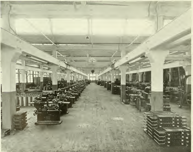
EXTERIOR AND INTERIOR VIEWS OF THE NEW HEALD ADDITION
