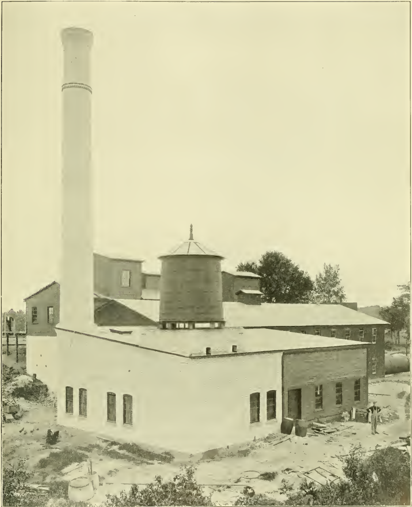
THE PLANT FROM THE RAILROAD SHOWING BOILER AND ENGINE HOUSE AND STACK
