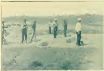
Laying Reinforced Concrete Pavement by the Hassam Paving Process
