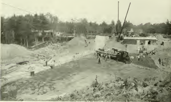
THE MONSTER 1400 FOOT DAM UNDER CONSTRUCTION AT KENDALL RESERVOIR
