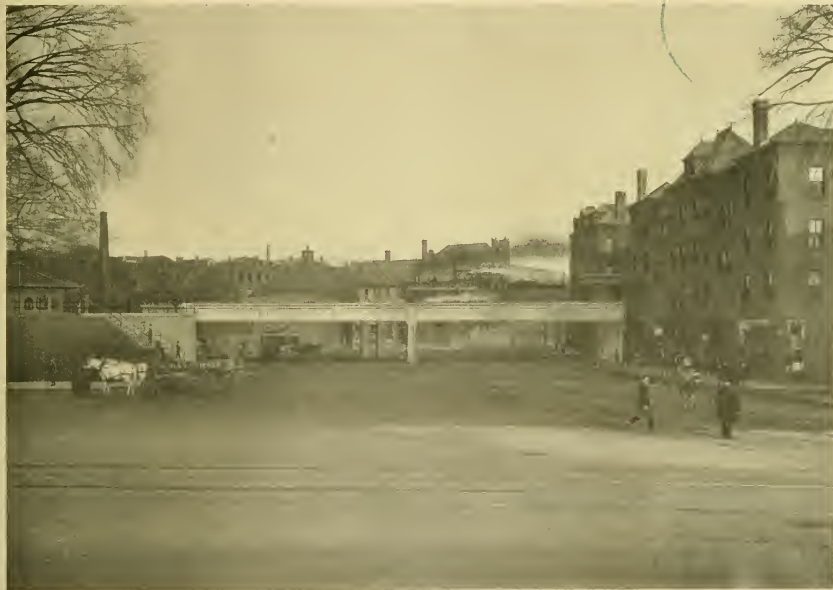
LINCOLN SQUARE WITH GRADE CROSSING REMOVED SHOWING TYPE OF BRIDGE, STEEL, FACED WITH CONCRETE; PROPOSED BY PROF. CHARLES B. BREED
