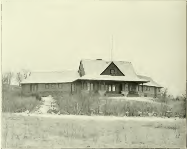
THE RANGE HOUSE LOOKING SOUTH FROM THE FIRING LINE
