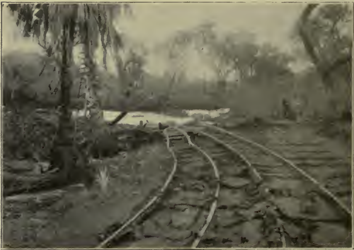
ONE OF THE TROLLEY LINES AFTER THE FLOOD.
