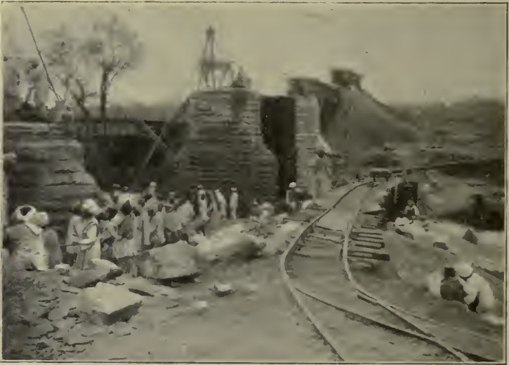
“THE HEAVY STONES WERE SWUNG INTO POSITION.”
