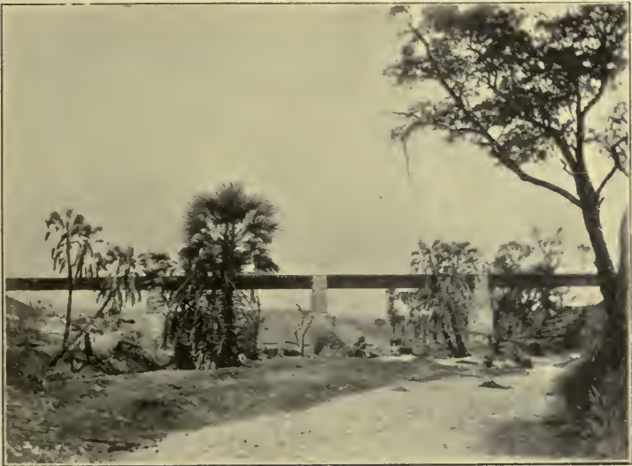
THE COMPLETED TSAVO BRIDGE.
