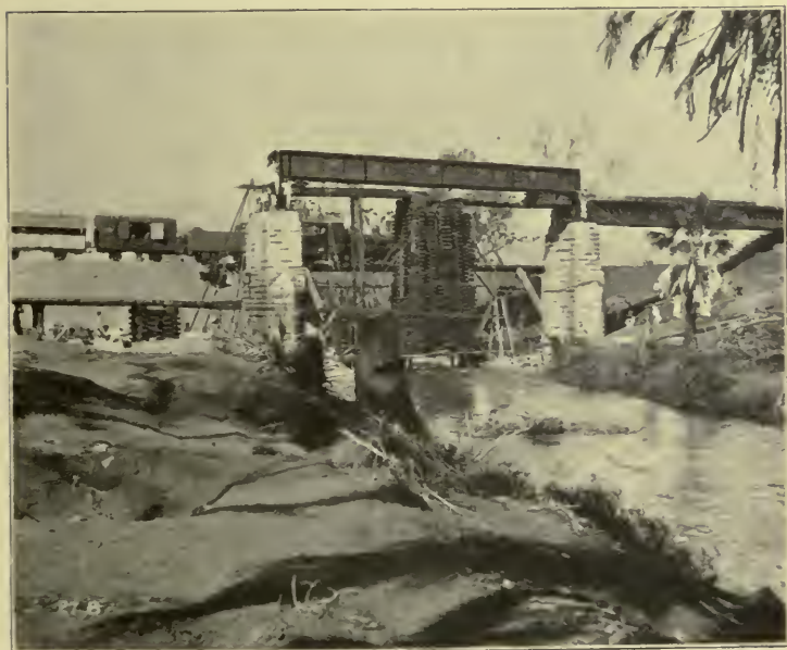
"AND FINALLY LOWERED GENTLY INTO POSITION."
