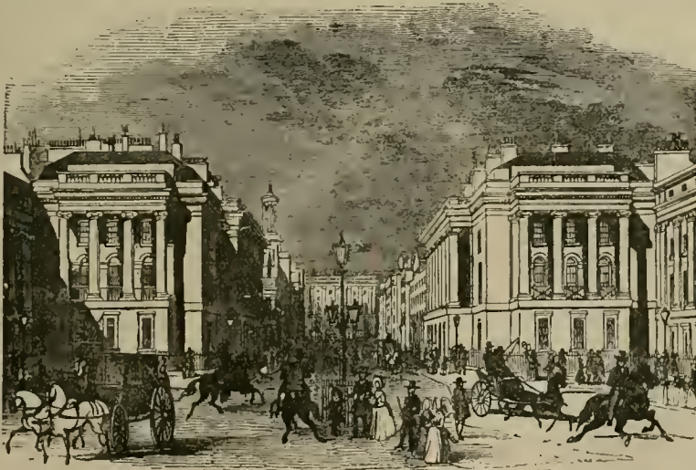
Waterloo Place, leading toward Regent-street.
