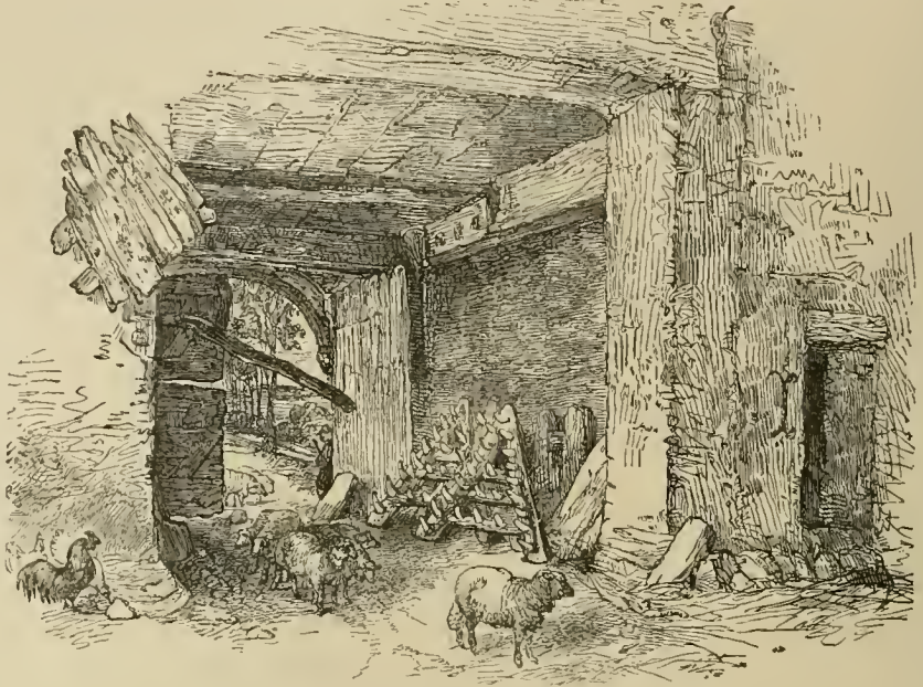
Hougoumont—Gateway of Farm-Yard, from the Interior.
