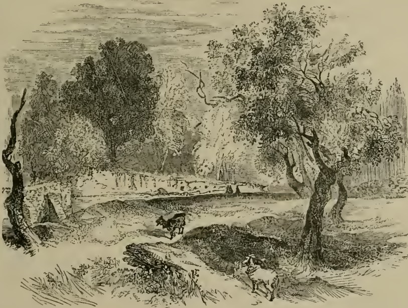
Hougoumont—Exterior of Garden Wall.
