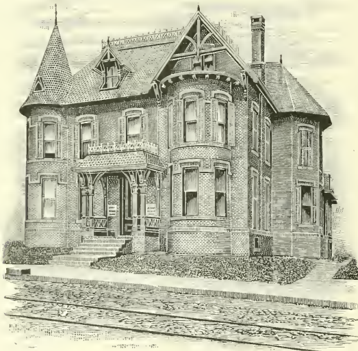
THE DIME SAVINGS BANK (REFERRED TO ON THE PRECEDING PAGE). ALSO THE OFFICE OF HOLMES & PARSONS, BANKERS. (SEE FURTHER, PAGE 178.)
