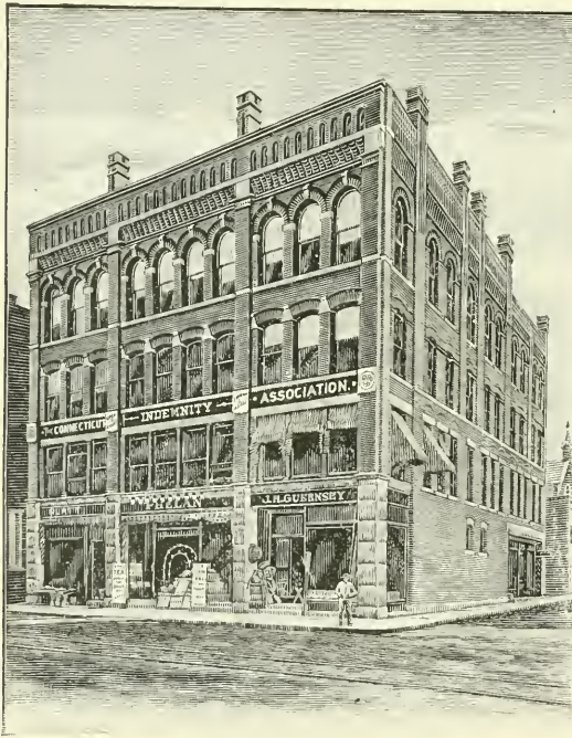
THE PLATT BLOCK, OFFICE OF THE CONNECTICUT INDEMNITY ASSOCIATION.
