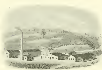
THE EAST MILL OF THE WATERBURY BRASS COMPANY, 1858.
