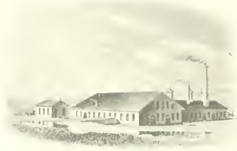
THE WEST MILL OF THE WATERBURY BRASS COMPANY, 1851.
