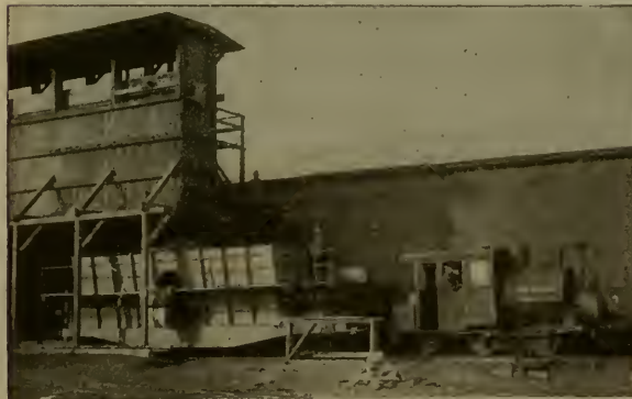
Distributor Car Taking Load of Mixed Feed, Capacity 20,000 Lbs.
