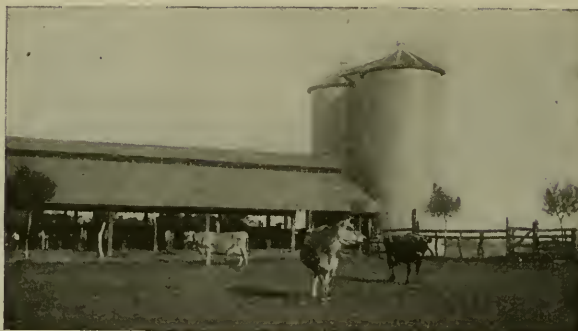
Dairy barn and silos, owned by Ed. C. Lasater, Falfurrias, Texas, in the land of sunshine, "The Land of Heart's Delight." The dairy barn is built so as to admit plenty of air. The cow animal, as well as the man animal, needs canned vegetables during the winter months. Hence, the Silo.
