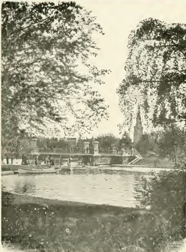
Boat and Bridge Scene Public Gardens
