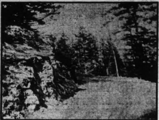
The above photographs show the construction of the road up the Saanich mountain, now being built by the provincial government. Upper is the first earth cut on the road near the point where it leaves the West Saanich road; lower is a typical rock cut. The road is almost half done, except for the metal surfacing, and the preliminary work is open for a considerable section further up. About 100 men are engaged.
