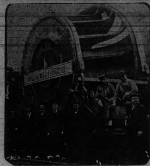
TURBINE FOR MUSCLE SHOALS. —This turbine casting, seventeen feet high, weighing seventy tons, is to become part of the gigantic power plant at Wilson Dam, Muscle Shoals. From the foundry at Wheeling, W. Va., to its destination the route was carefully calculated and tunnels measured to avoid those that were too small.
