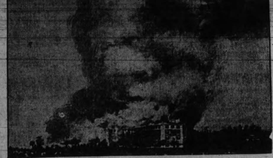
PALM BEACH'S $2,000,000 FIRE The Breakers, fashionable hotel at Palm Beach, Fla., at the height of the fire which destroyed it and other property, causing heavy losses to rich guests and local property owners.
