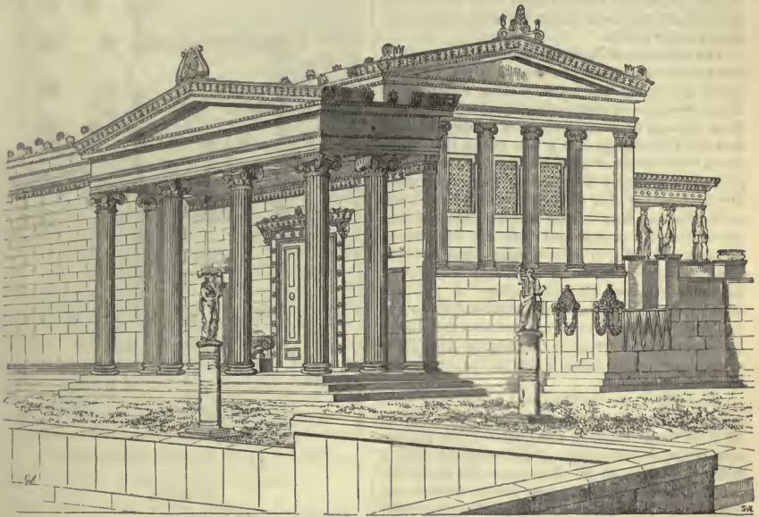
THE ERECHTHEIUM RESTORED, VIEWED FROM THE NW. ANGLE.
