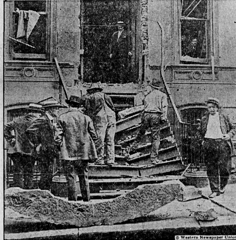
A photograph of the residence of Judge Charles C. Nott, Jr., in New York city, which was partly demolished by a bomb placed in the vestibule by an unknown person. The explosion, which shattered every window in the immediate neighborhood, shook the section for miles around. One person, a watchman, was killed. This was part of the anarchist bomb plot in eight cities of the East.
