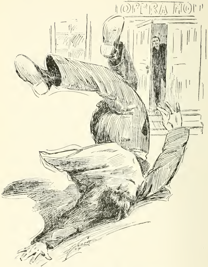
"Struck on his head in front of the building."
