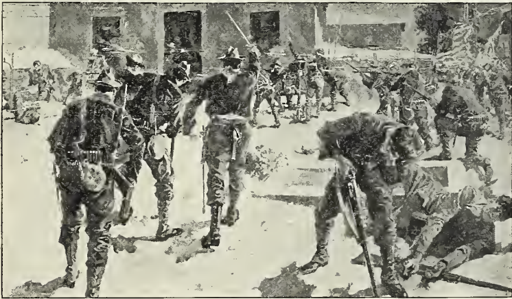
Capturing the Spanish Block-house, San Juan.
