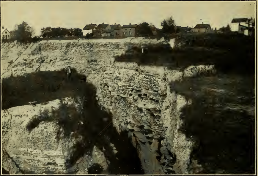
FIGURE 1.—THE FISSURE FROM THE TOP OF THE CLIFF
