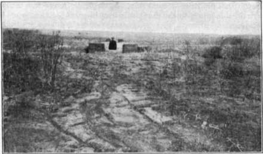
FIG. 22.—Stop plank dams built in terrace outlet channel at ends of graded terraces to prevent the erosion of a gully down through the field. Note the sediment above the dam. A gully which formerly existed along the line of the stop plank dams has been completely filled up.
