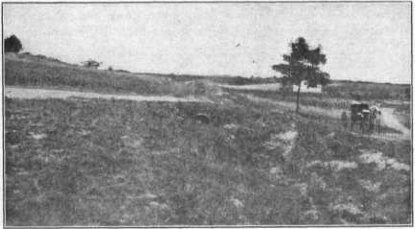
FIG. 38.—Method of carrying terrace water under a roadway by means of a culvert.
