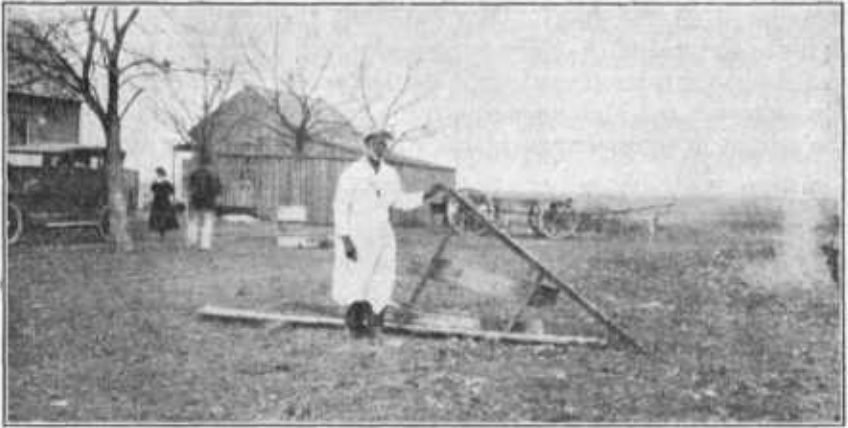
FIG. 32.—View of homemade wooden V drag used for throwing up terraces.
