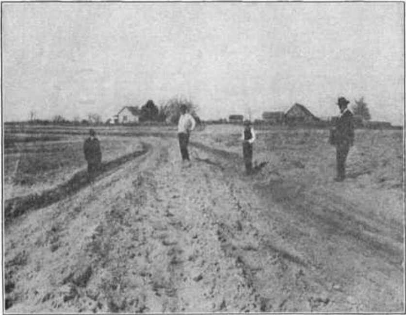
FIG. 35.—View of a newly completed broad-base ridge terrace.
