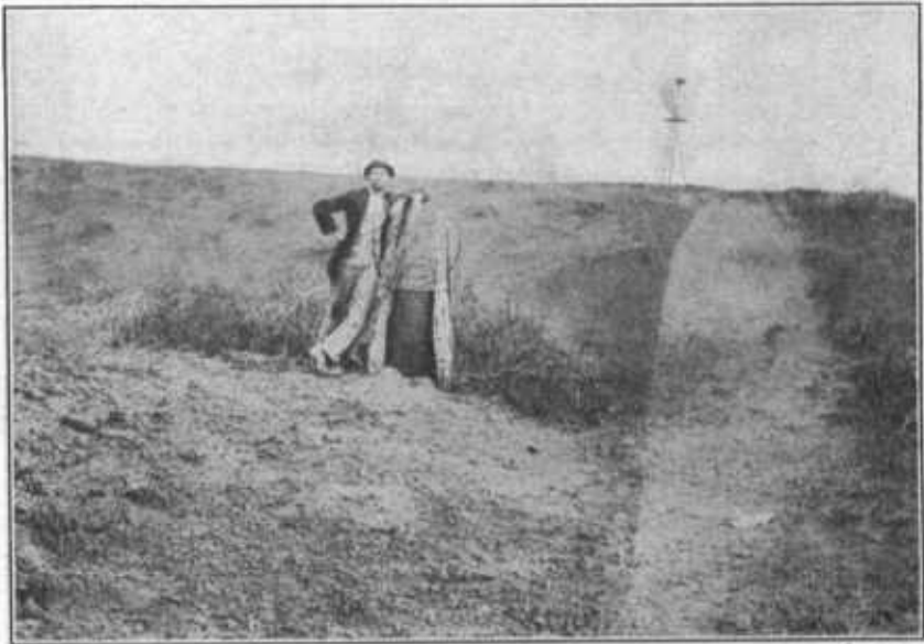
FIG. 26.—Upper side of newly constructed soil-saving dam, showing inlet pipe.
