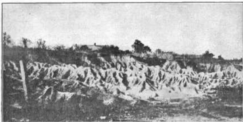
FIG. 5.—Erosion chiefly caused by alternate freezing and thawing followed by heavy rains.
