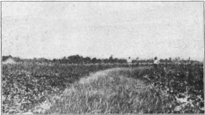
FIG. 37.—Newly built terrace seeded to cover crop to insure against breaking before the loose earth becomes thoroughly settled.
