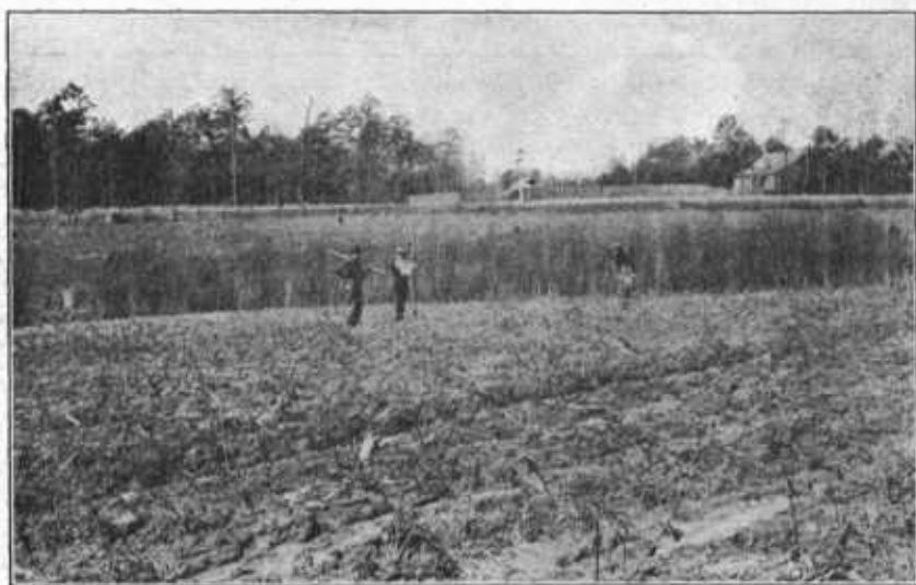
FIG. 30.—View showing a party laying off terraces. The man with hoe digs a hole at each position of the rod to guide the plowman in laying out the first furrow of the terrace.
