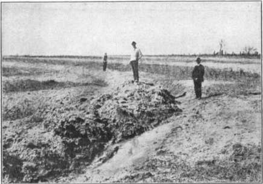
FIG. 36.—High terrace embankment built across a draw with a slip scraper.
