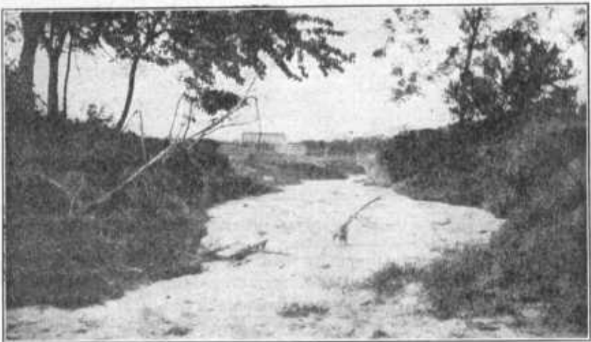
FIG. 3.—Drainage ditch partly filled with sand washed from eroding hills.
