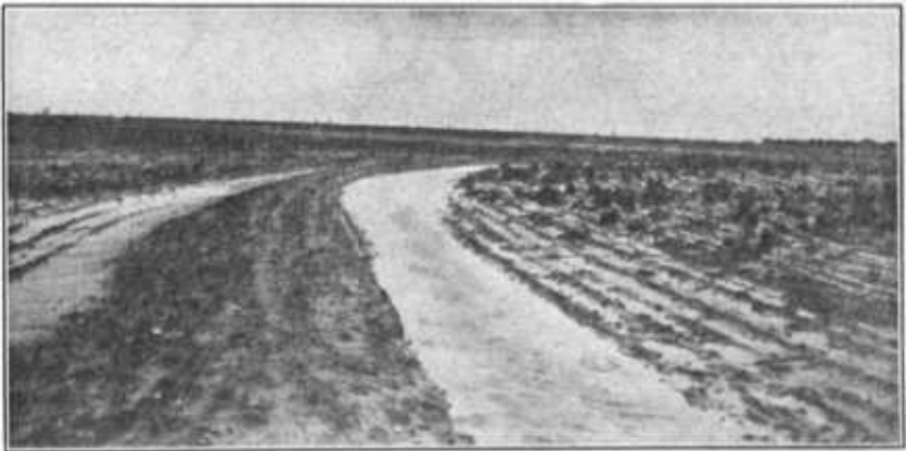
FIG. 19.—View showing water flowing off in a broad shallow channel of a broad-base graded ridge (terrace). (From Bulletin B-23, A. & M. College of Texas.)
