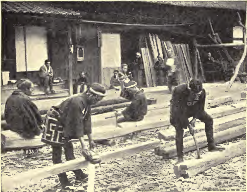
CARPENTERS AT WORK
