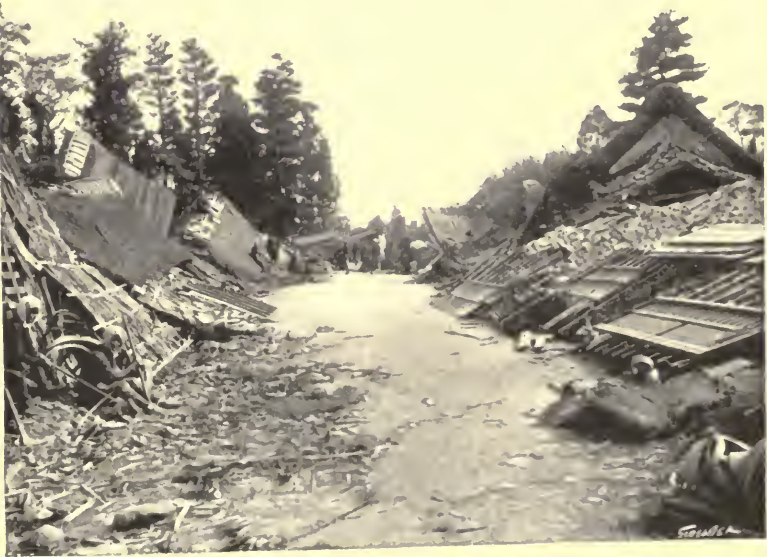
RESULTS OF THE EARTHQUAKE
