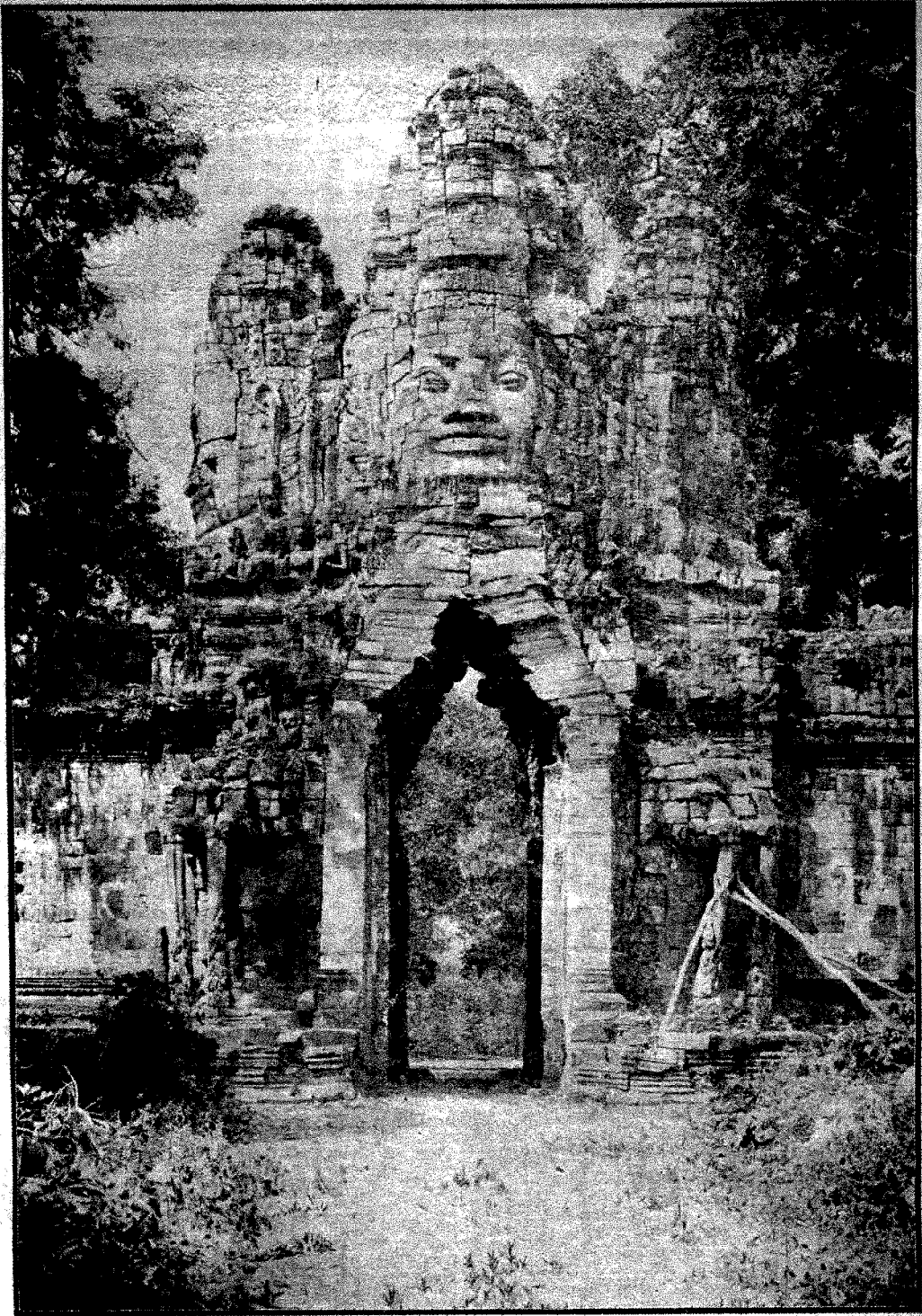
Angkor-Thom—North gate surmounted with the four heads of Brahma. It is to be noted that the heads have been constructed with bricks of different shapes and sizes dexterously and judiciously put together.
