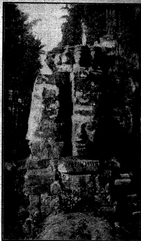
Angkor-Thom—Ornamental heads of Brahma. The heads have been constructed with bricks of different shapes and sizes judiciously put together.
