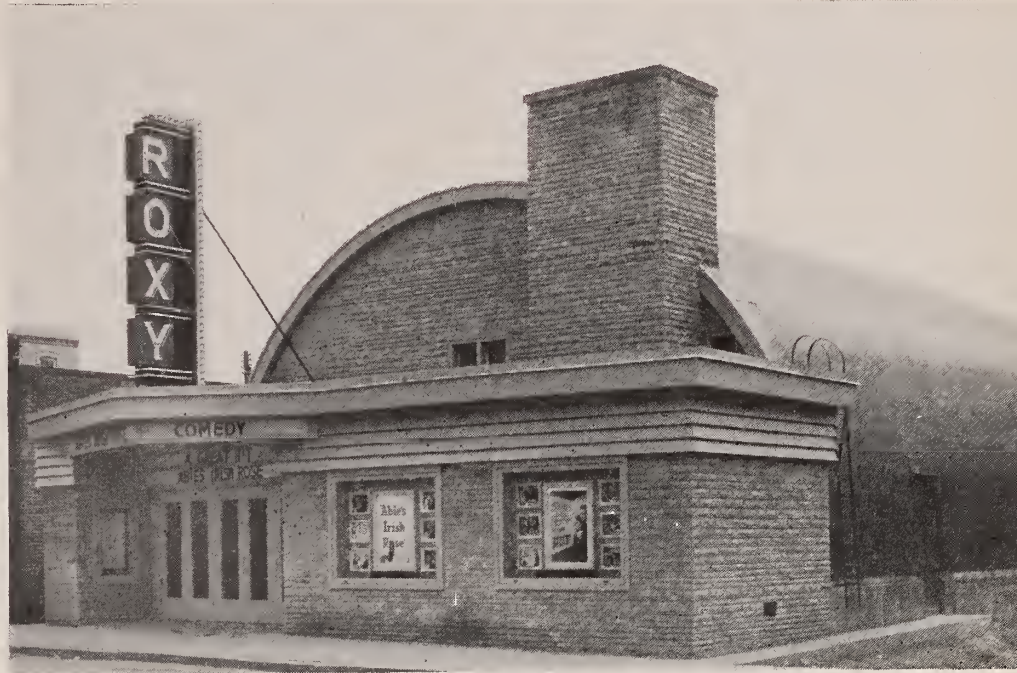
With a depth of 144 feet, 132 feet are of Quonset construction.
