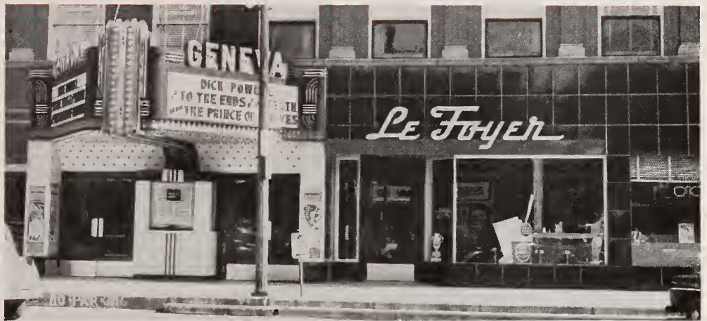
Front view of the new sandwich shop in the Geneva theatre.
