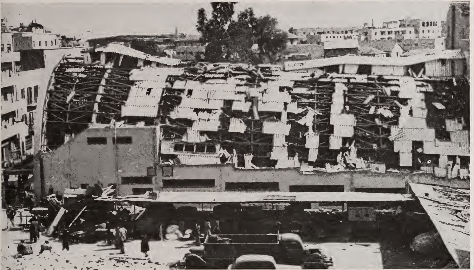
"The blast blew the roof off the theatre, crumbling partitions and shattering windows."
