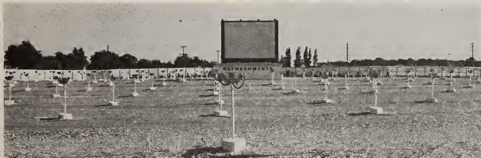
Broad acres of DeVry in-car speakers in the drive-in theatre near Muncie, Ind. Projectors and sound system are also DeVry. The Muncie drive-in accommodates 750 cars and has a picture width of 42 feet, with a projection throw of 235 feet.
