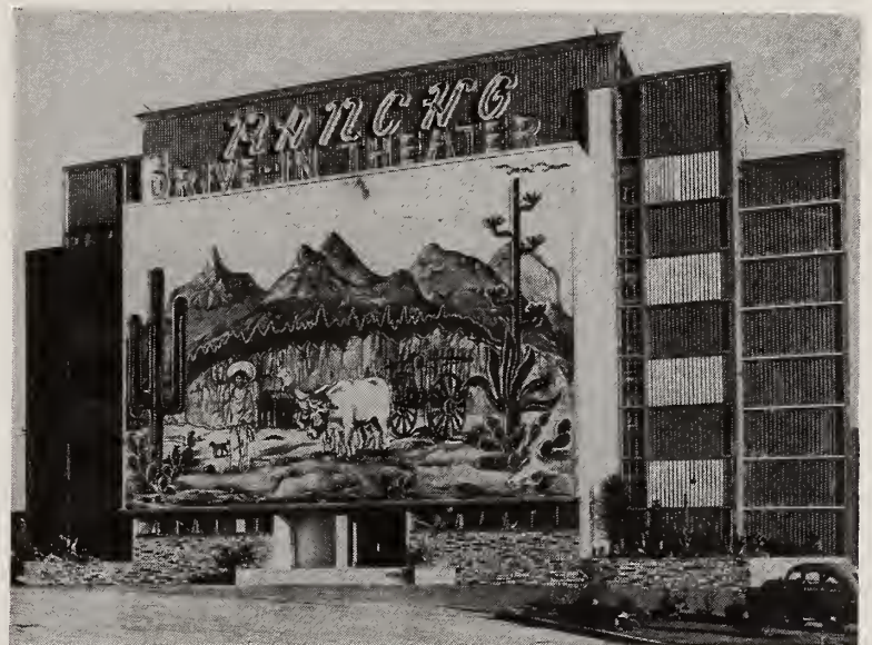
Entrance side of the Rancho screen tower, with its illuminated mural.
