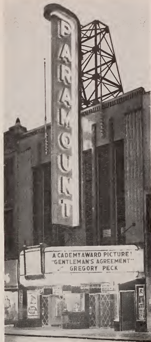
Built in the 1920's, lavish in its period design, the Paramount theatre in Rochester, N. Y., seating over 2,000, was one of many costly houses erected to glorify the motion picture and, like them, became obsolete and a problem of modernization. Pictured here are the results of its remodeling, for which Michael J. DeAngelis, Syracuse, was the architect.
