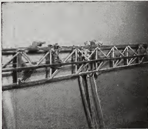
Setting up for mechanical screen resurfacing (above). The track starts at top and carries the spray gun (see detail view below) across the screen in downward steps.
