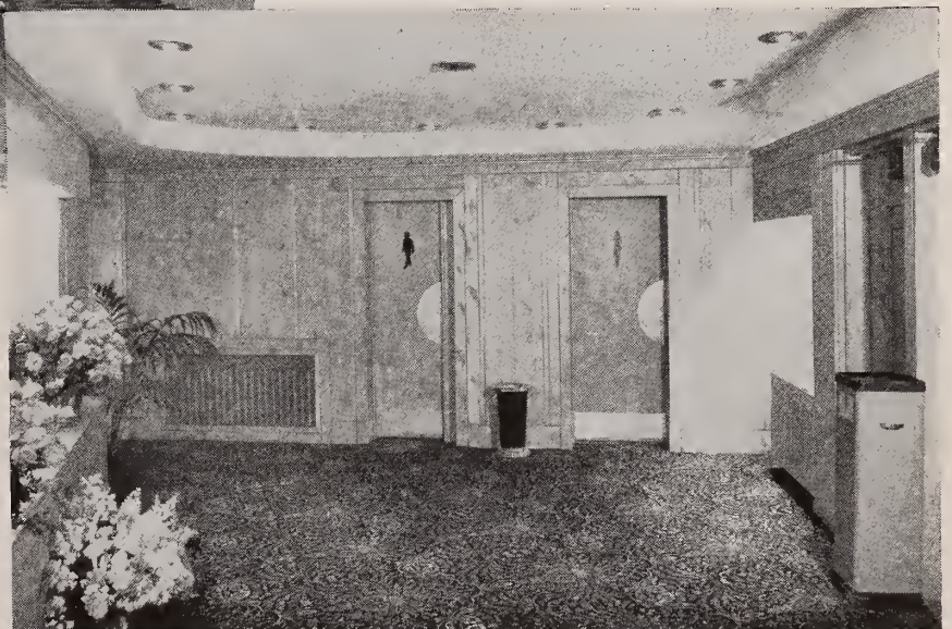
Looking across lobby toward toilet room doors.
