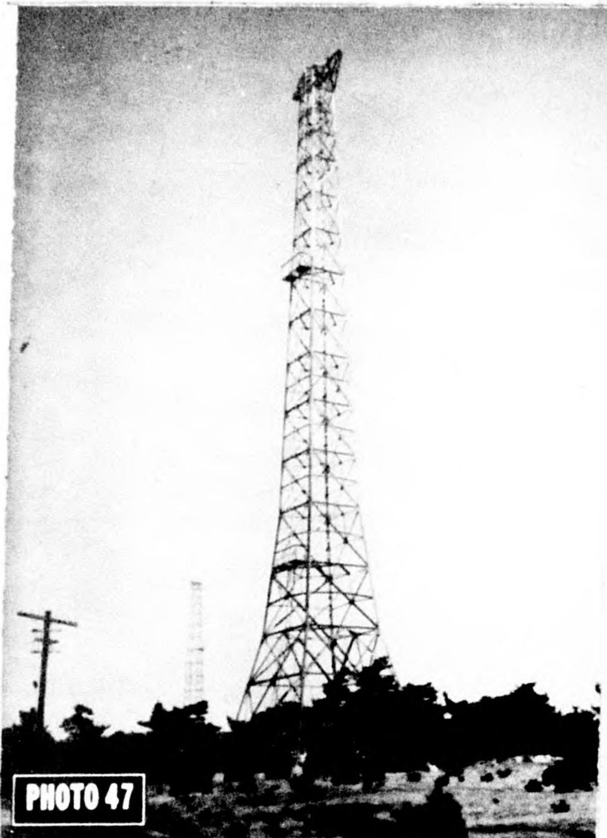
Lattice mast, near Fukuoka
