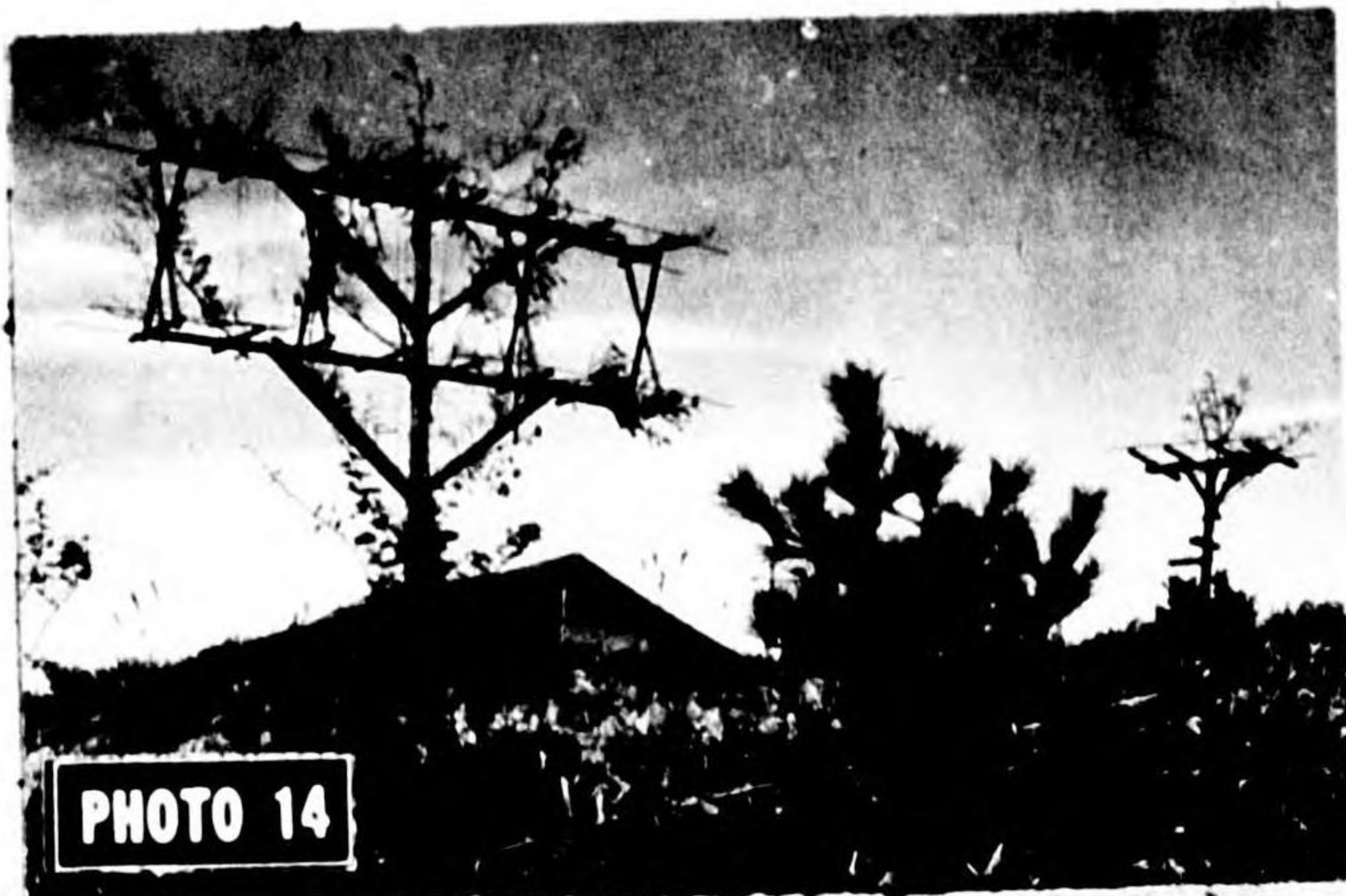
TACHI 6 Receiving antenna - Fukuoka region
