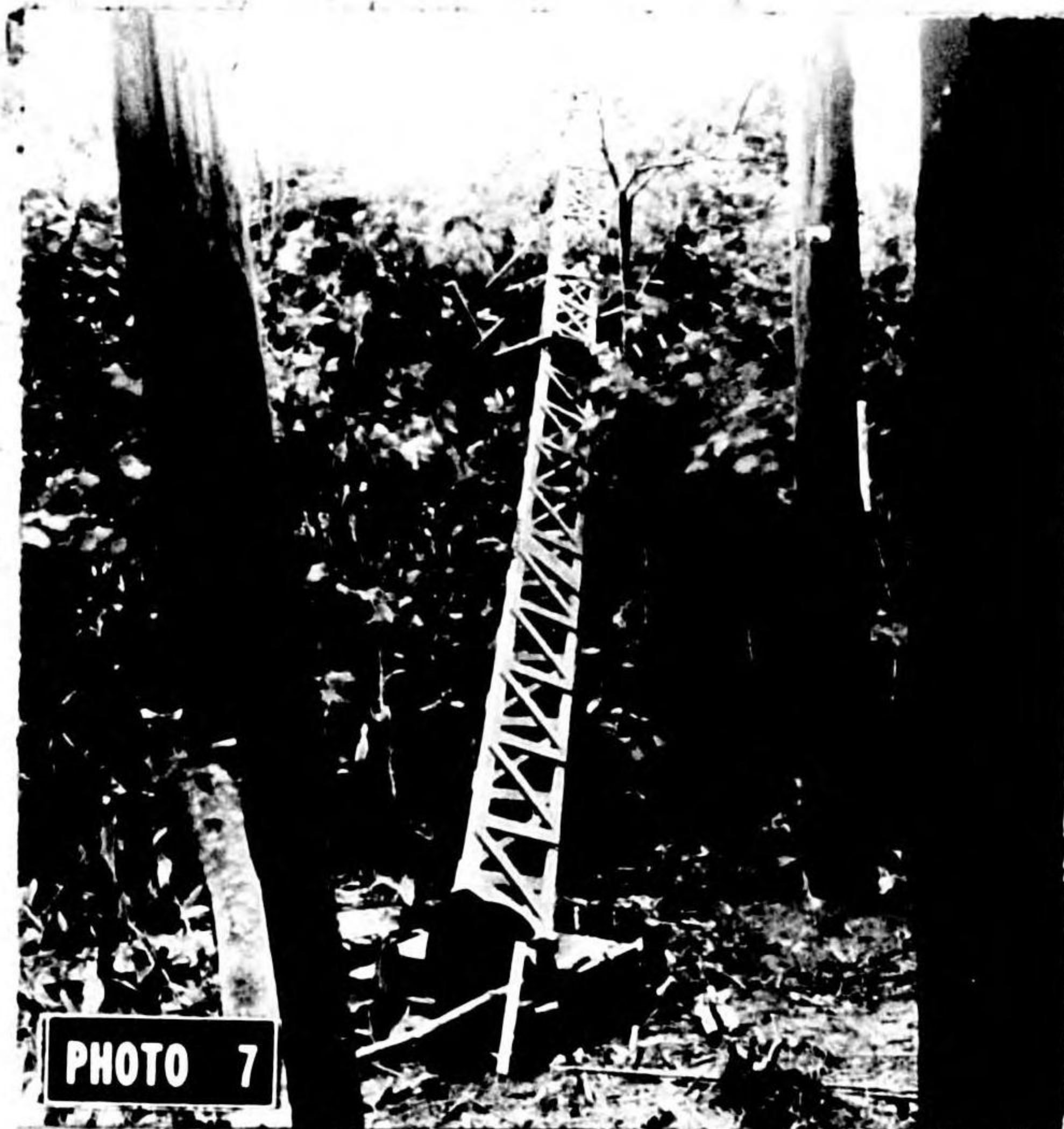
PHOTO 7 MK 13 Antenna - Damaged by Japs
