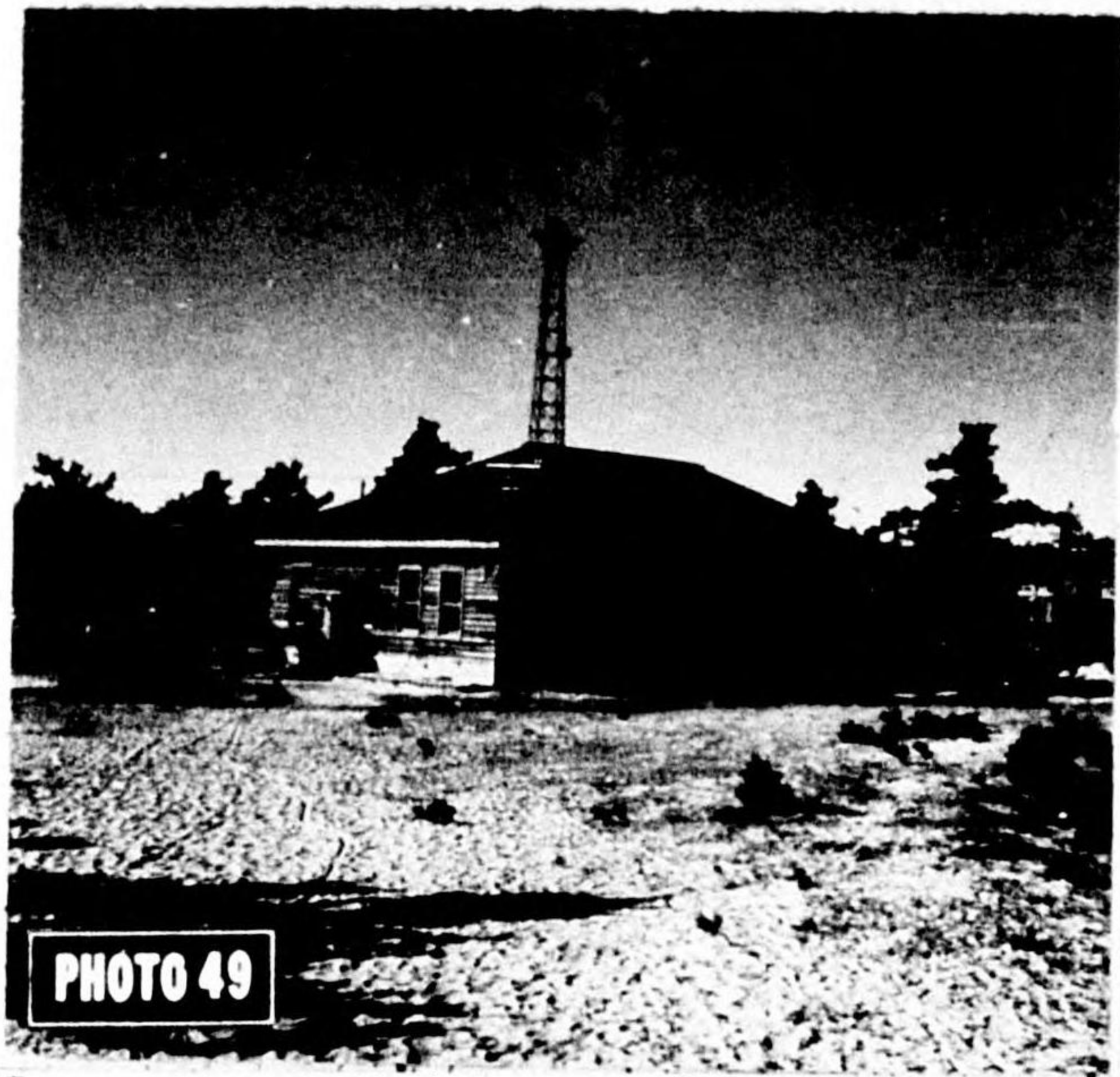
Transmitter building, near Fukuoka
