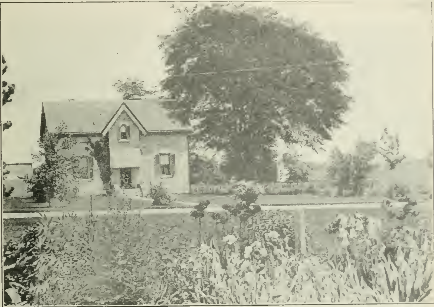
Fig. 4. Beneath the Elm tree's shade.
