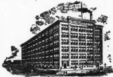
FACTORY 132 ND TO 133 RD ST & BROOK AVE
