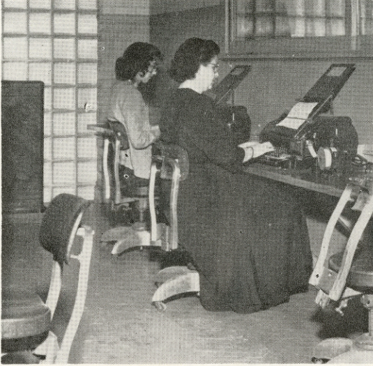
Six perforators cut tapes on locally written stories and want ads for use on teletypesetters.
