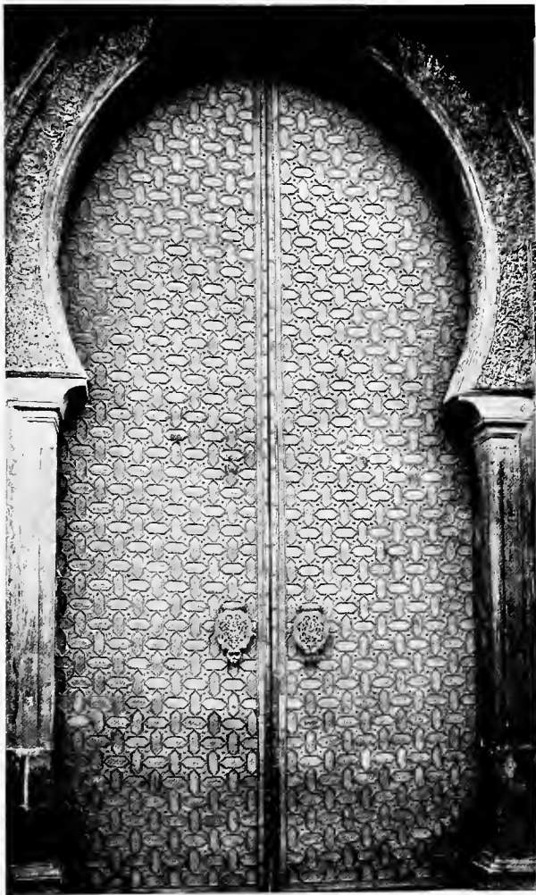
FIG. 10. COPPER-PLATED DOORS. Puerta del Perdón, Mosque of Córdoba. 1377.
