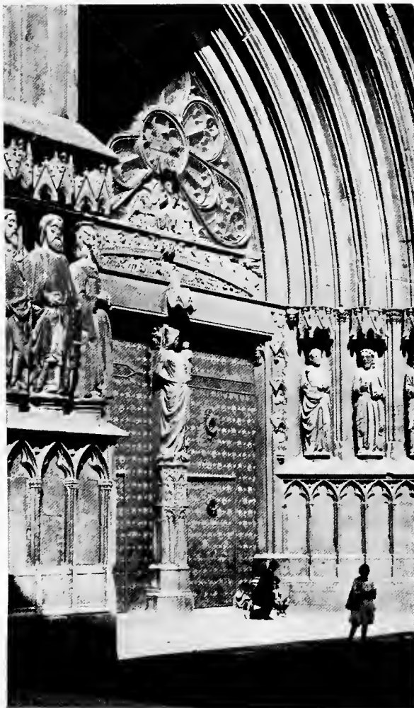
FIG. 13. IRON-PLATED DOORS. Main Portal of Tarragona Cathedral. 1510.
