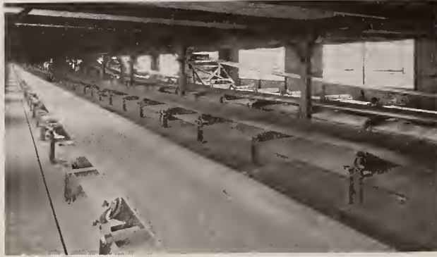
IN ONE OF THE CONVEYOR GALLERIES
