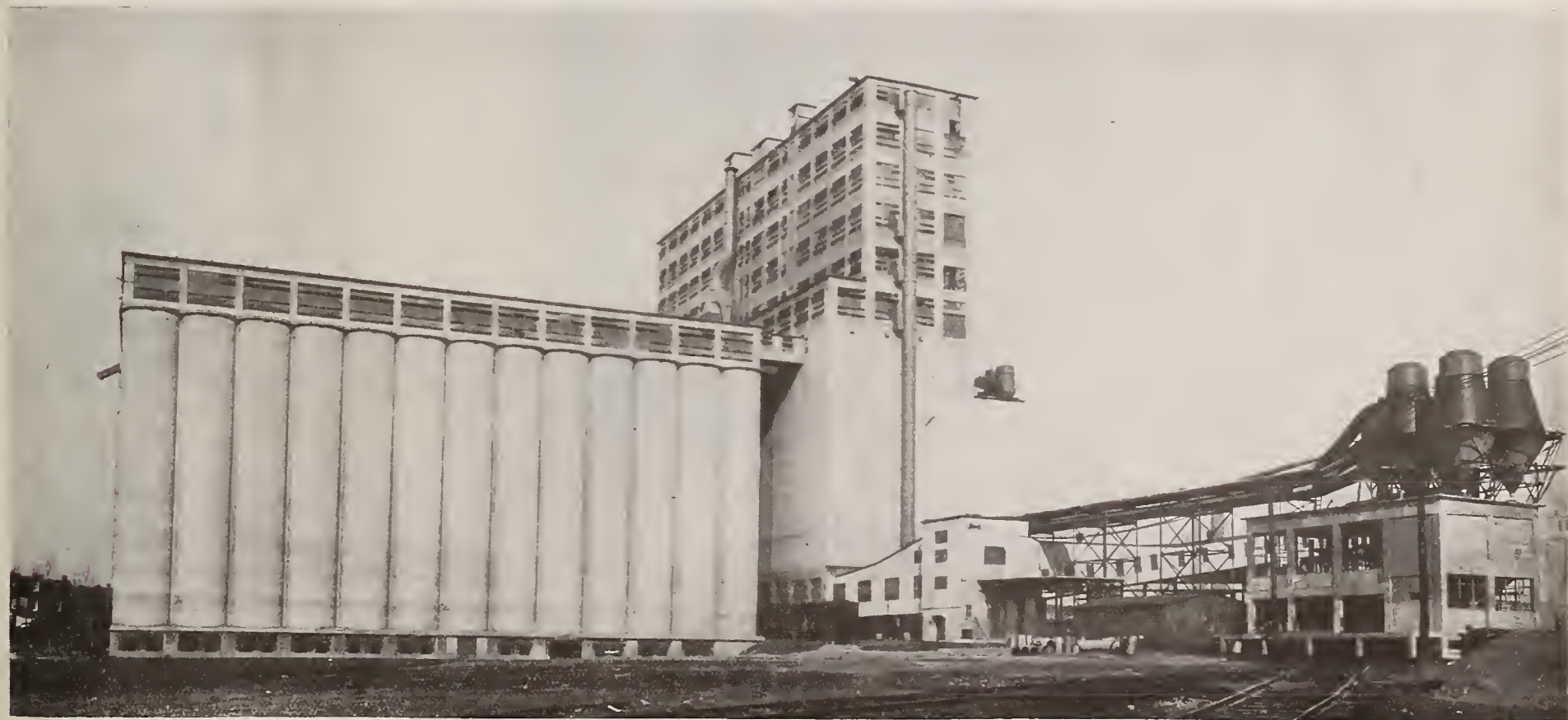
THE NEW BALTIMORE & OHIO ELEVATOR, LOCUST POINT, BALTIMORE, MD.
