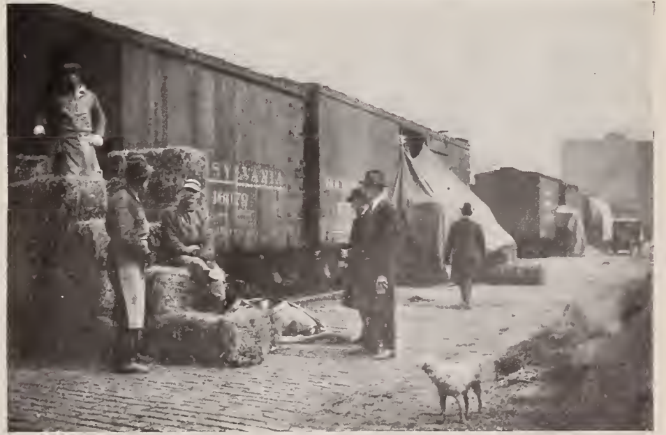
PROSPECTIVE BIDDERS MAKING AN INSPECTION
