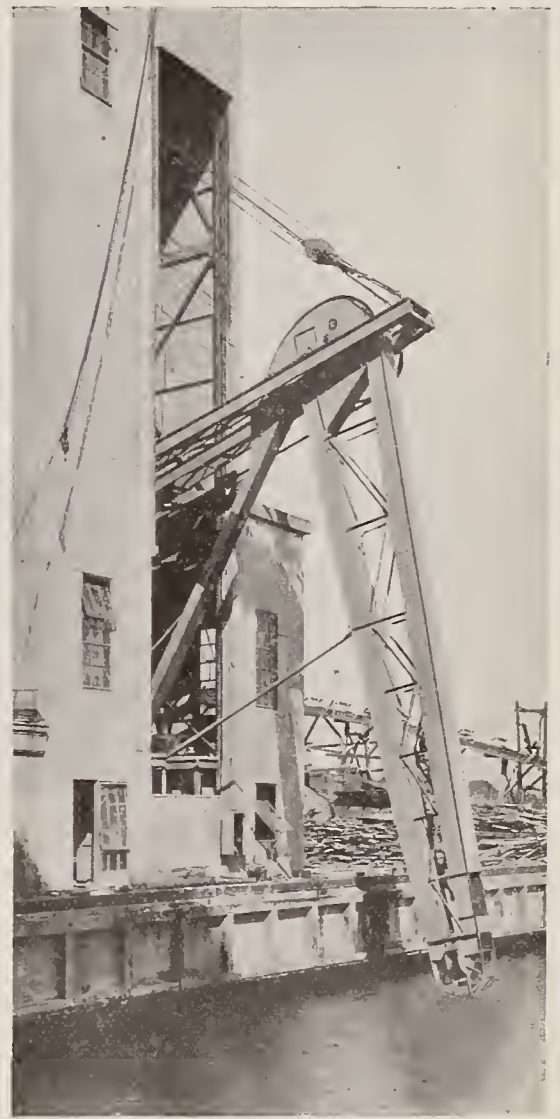
MARINE LEG PENNSYLVANIA RAILROAD ELEVATOR BALTIMORE, MD.
