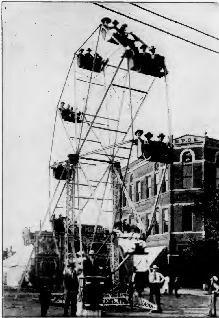
The above is a half-tone of the Big Eli Wheel built by the Eli Bridge Co., of Roodhouse, Ill., and featured with the New Parker Amusement Co. this season. This wheel proved one of the surprises and hits of the Great Dallas, Texas, Fair last fall. It is equipped with a truck which loads the entire wheel and seats, and to look at the big structure while in operation one would never think it could be gotten in so small a wagon. However, that is part of the business of the Eli Bridge Co. Its new factory at Roodhouse has been crowded all season and is still far behind on orders for structural work. Within another year this progressive firm will build another large fire proof factory to accommodate its rapidly increasing business.
