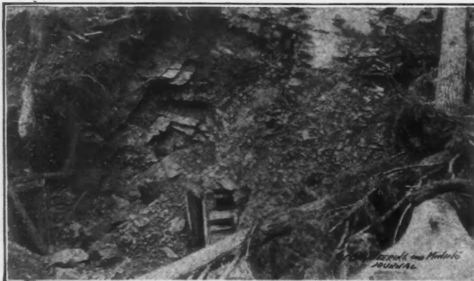
FIG. 1. DISCOVERY TUNNEL OF THE ANTHRACITE FIELD IN MT. BAKER DISTRICT
