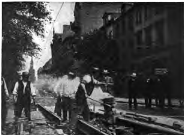
WELDING STREET RAILWAY TRACKS BY THE THERMIT PROCESS.
