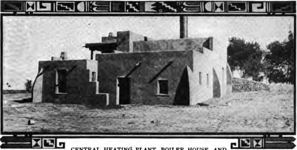
CENTRAL HEATING PLANT, BOILER HOUSE, AND FUEL BINS, ALL BUILT ON PUEBLO LINES.
