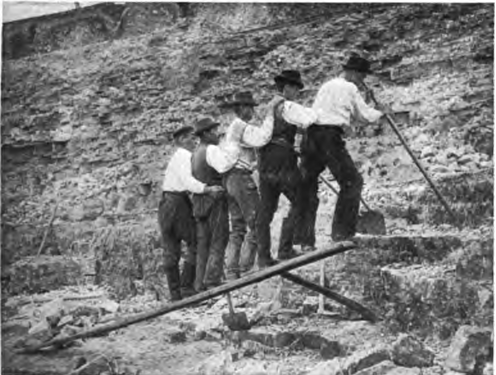
TILTING CROW-BAR FOR REMOVAL OF STRATIFIED QUARRIES.
