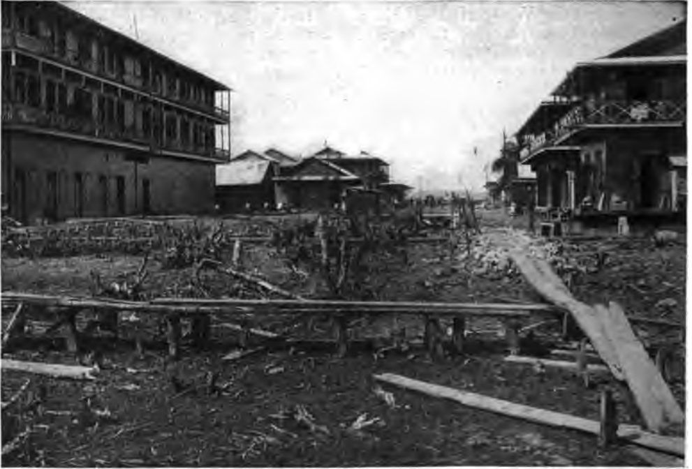
TENTH STREET, COLON, BEFORE PAVING
