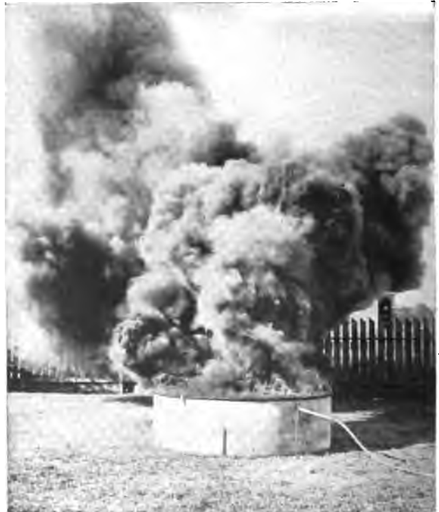
EXPERIMENTAL OIL FIRE EXTINGUISHED IN TWENTY SECONDS AT A COST OF THIRTY-FIVE CENTS.
