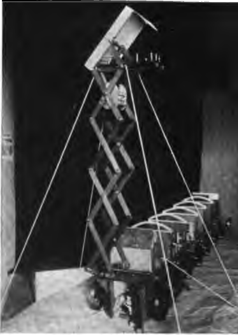
BIVOUAC CAR EXTENDED, WITH WALL AND ROOF REMOVED AND TOWER ERECTED.
