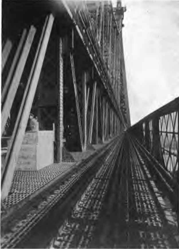
RAPID TRANSIT TRACKS OVER THE QUEENSBORO BRIDGE.
