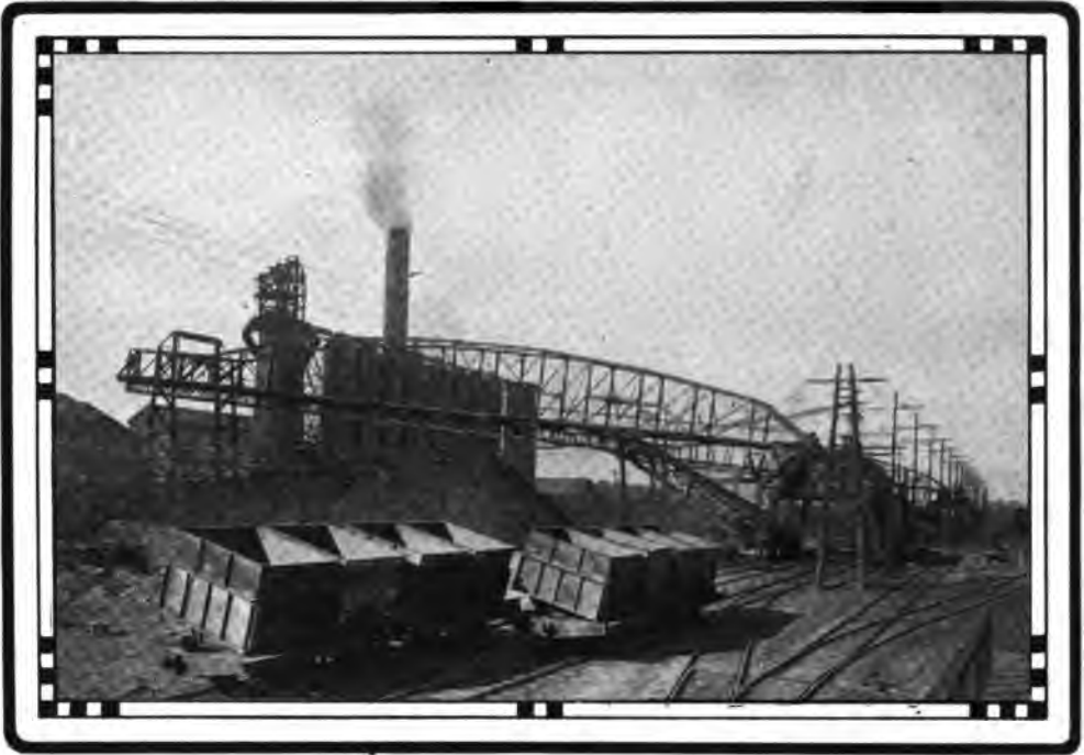
ORE HANDLING APPARATUS AT BLAST FURNACE.
