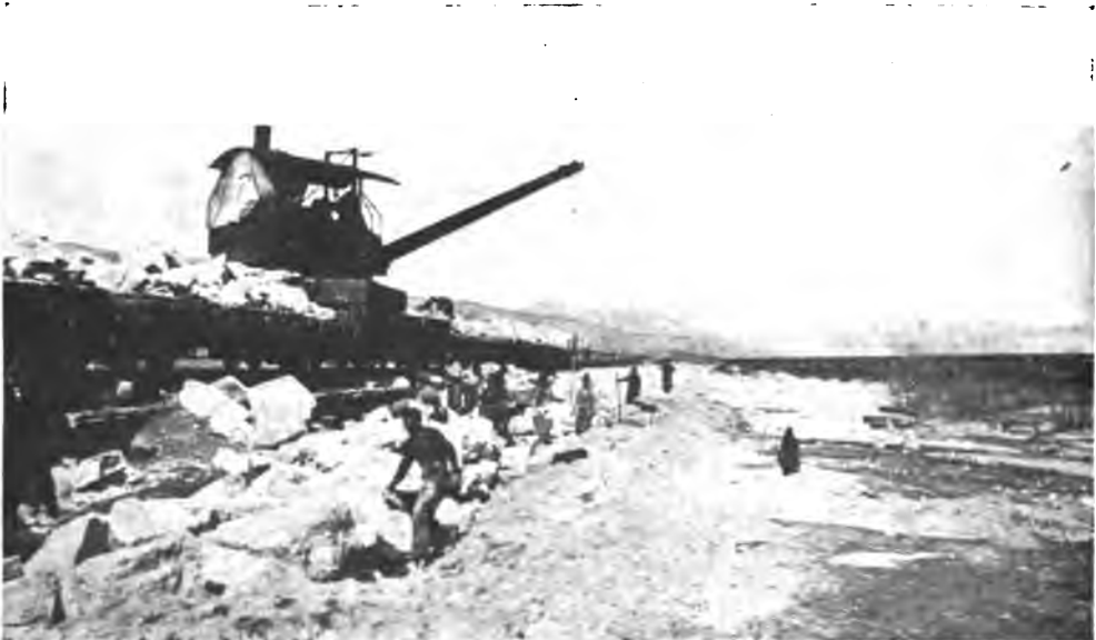
LAYING THE HALF-TON ROCKS OF THE HEAVY BULKHEAD IN PLACE.
