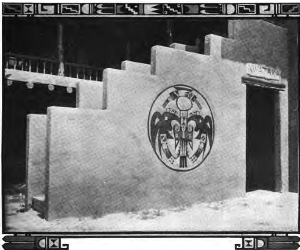
STEPS LEADING UP INTO KWATAKA—THE MEN'S DORMITORY.
