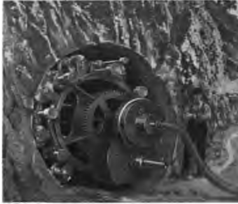
THE ROTARY TUNNEL MACHINE AFTER IT HAS WELL EATEN ITS WAY INTO THE ROCK. The hose carries the water required in drilling to the face of the drift.
