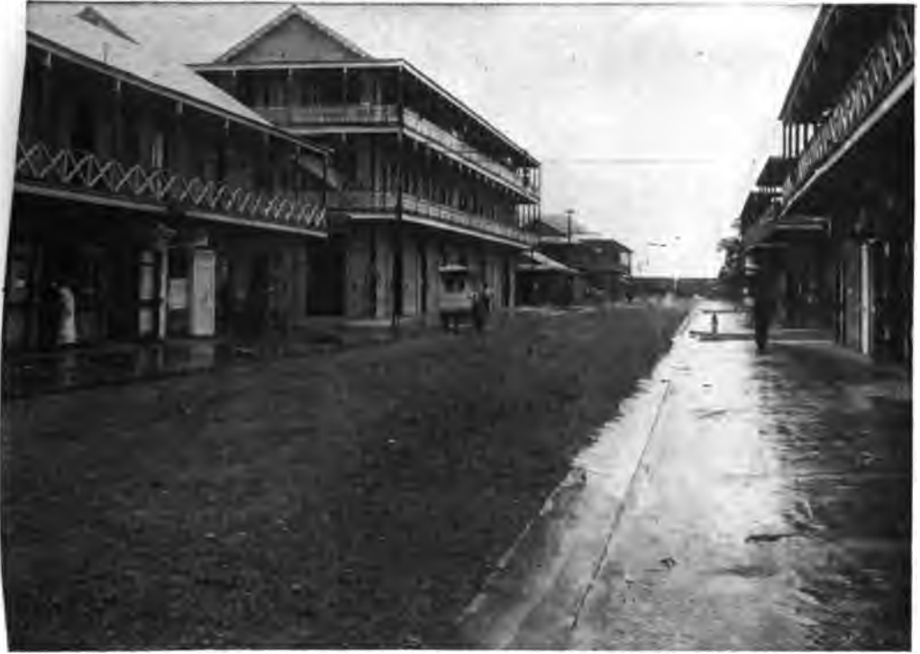
TENTH STREET, COLON, AFTER PAVING.
