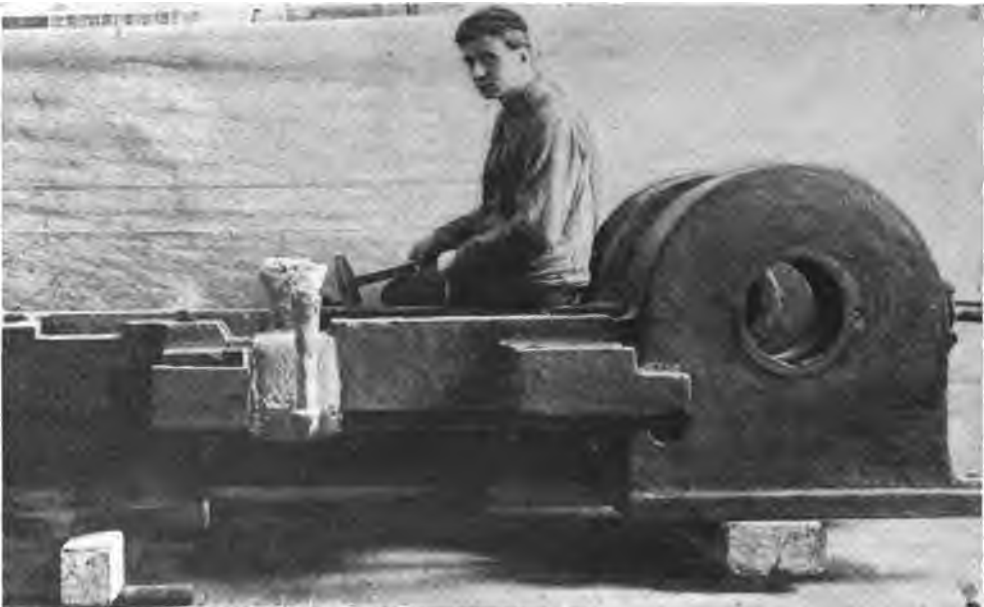
CAST-IRON SCREW-PRESS REPAIRED WITH RING OF THERMIT.
