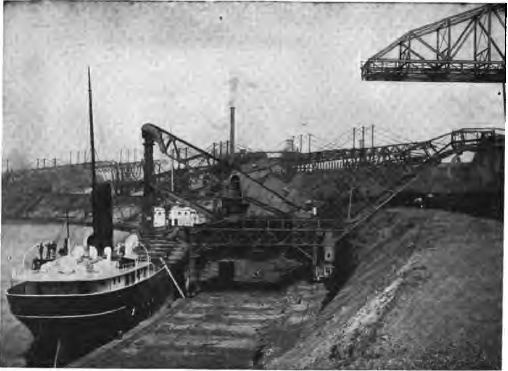
UNLOADING ORE FROM VESSELS AT THE DOCKS. WITH AN ELECTRIC CRANE.
