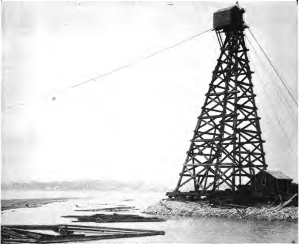
A CLOSER VIEW OF A SECTION OF THE COFFERDAM.
