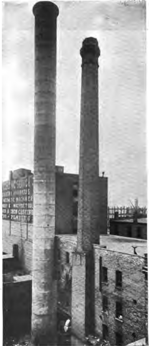
AN ENORMOUS STACK OF REINFORCED CONCRETE.
