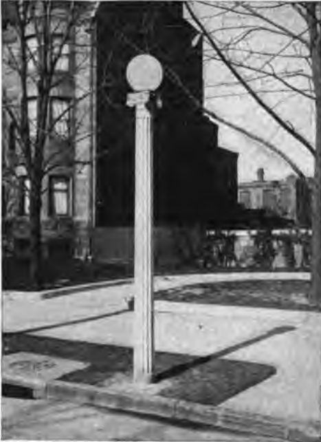
EXPERIMENTAL CONCRETE LAMP POST.
