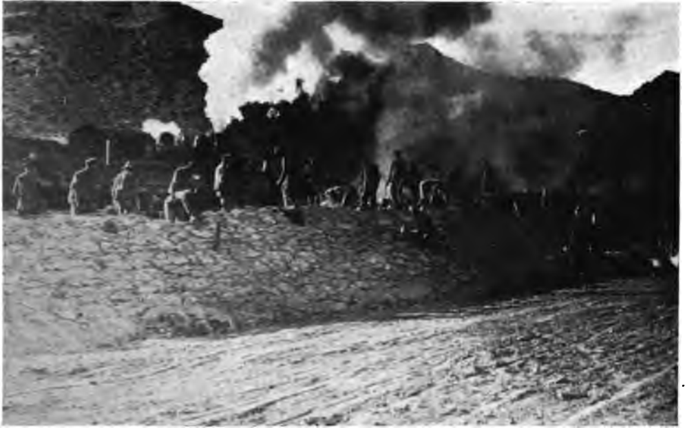
MILES OF RIPRAP LAID BY HAND ALL THROUGH THE MEADOW VALLEY WASH. Probably the most carefully constructed piece of roadbed in all the West.
