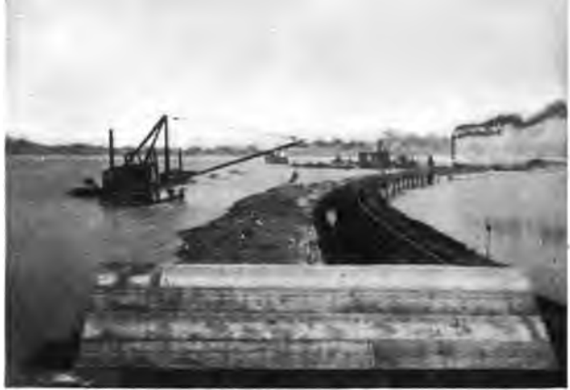
SECTION OF COFFERDAM BEFORE IT WAS TIMBERED OUT.
