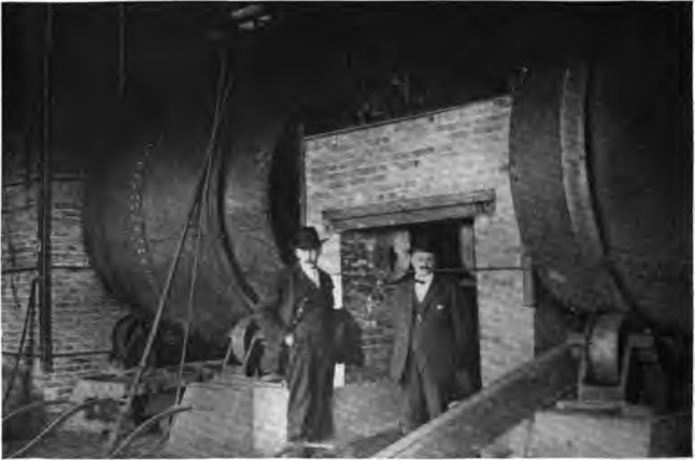
THE ROTARY CYLINDERS AND THE CONNECTING CHAMBER OF THE FINK SMELTER.
