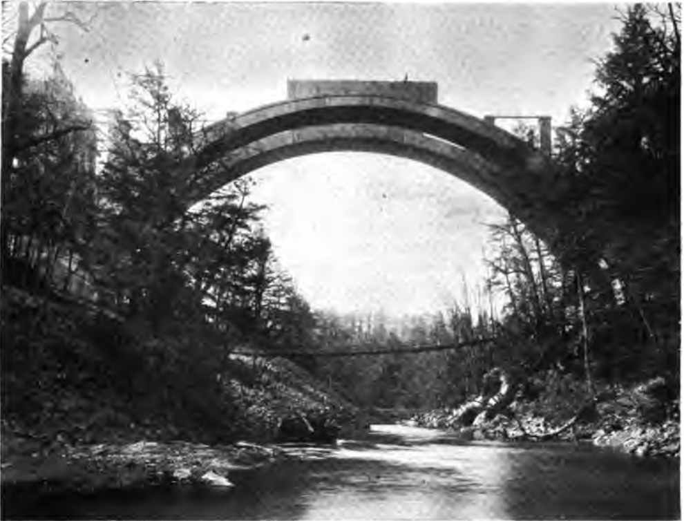
TWO BIG ARCHES. FREE OF CONCRETE MOULDING FRAME-WORK. FORMING PART OF WALNUT LANE BRIDGE.
