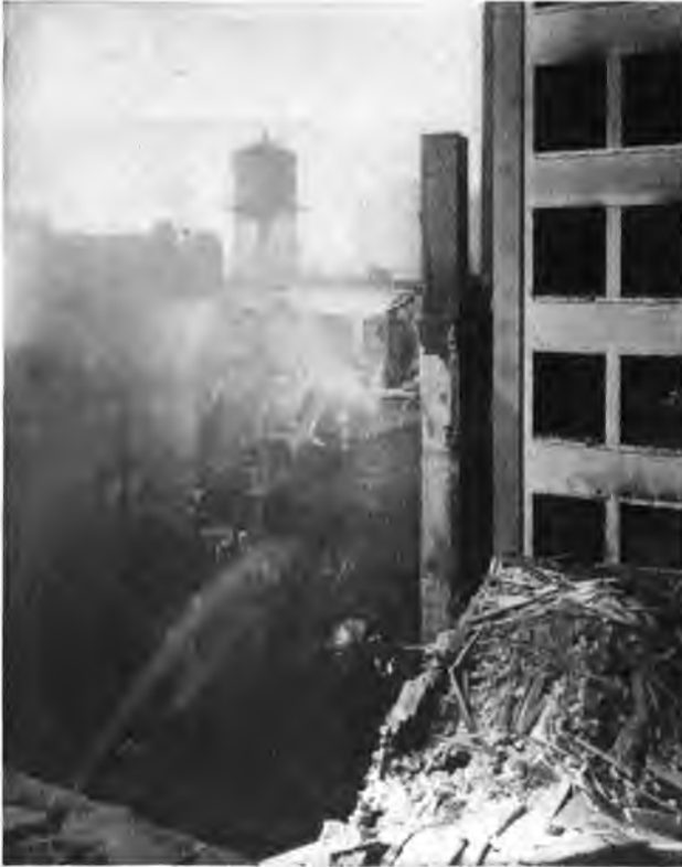
A FIRE IN THE HEART OF DOWNTOWN CHICAGO. Fortunately the adjacent buildings were really fire-proof.
