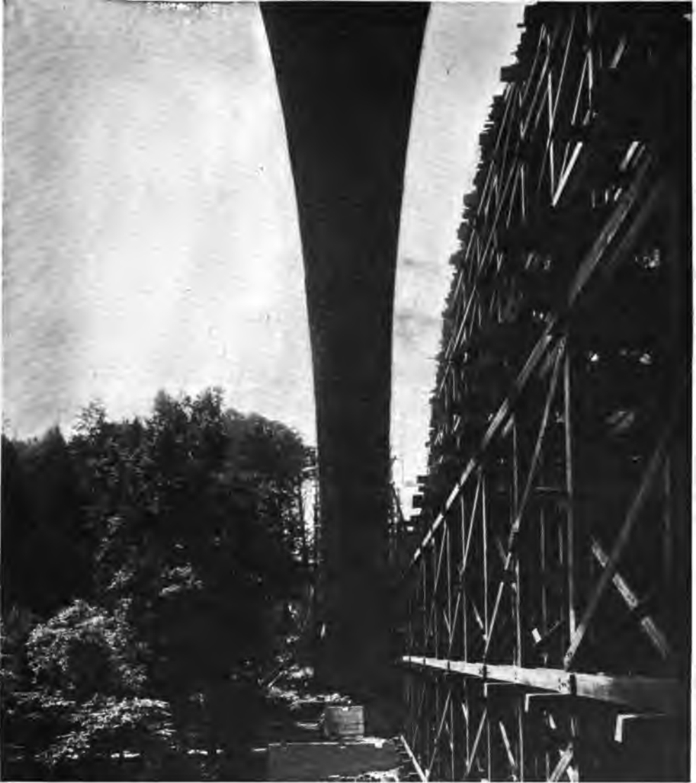
WALNUT LANE BRIDGE. PHILADELPHIA.
