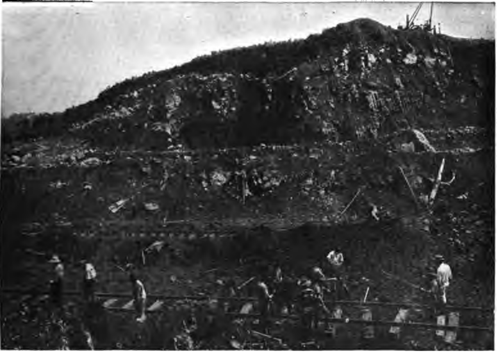
WAY AT GATUN. dam of that name is being constructed
