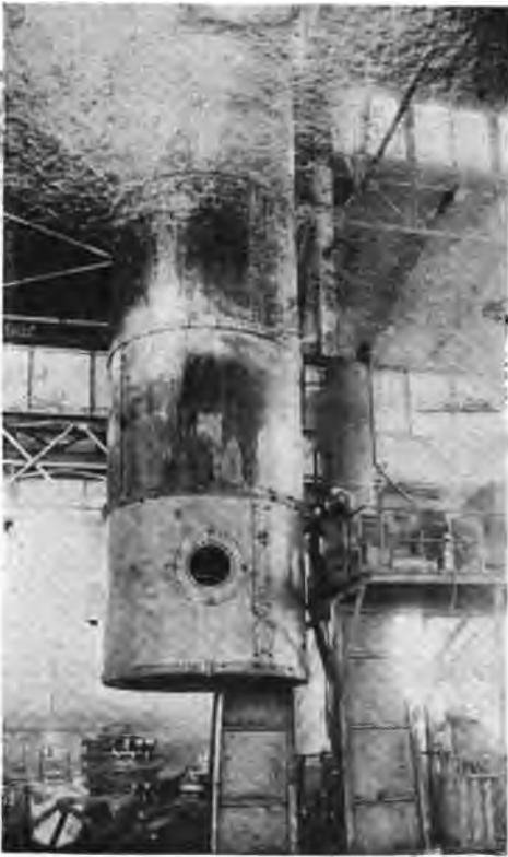
A SECTION OF THE GREAT NIAGARA FALLS PENSTOCK.
