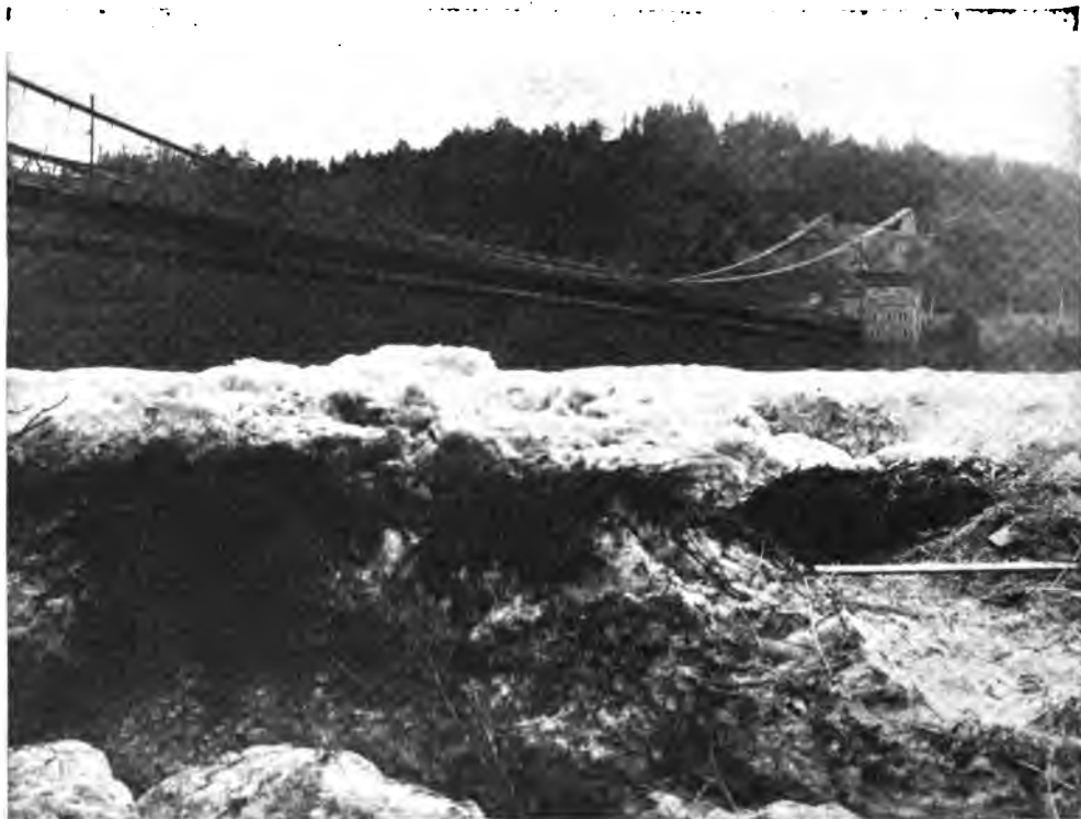
LEWISTON SUSPENSION BRIDGE ENDANGERED BY ICE-JAM This bridge is 65 to 85 feet above river at normal.
