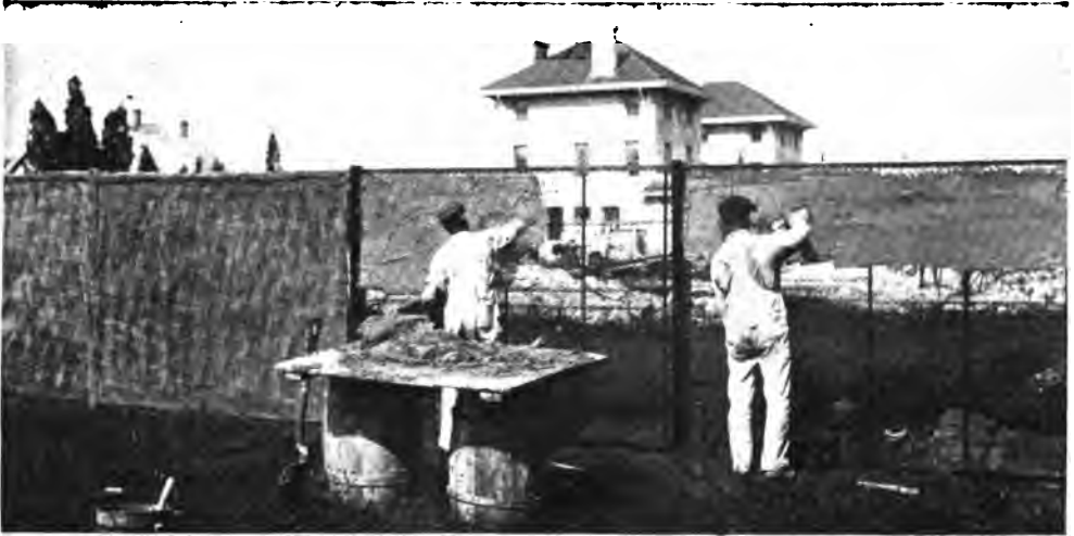
BUILDING A CONCRETE FENCE.
