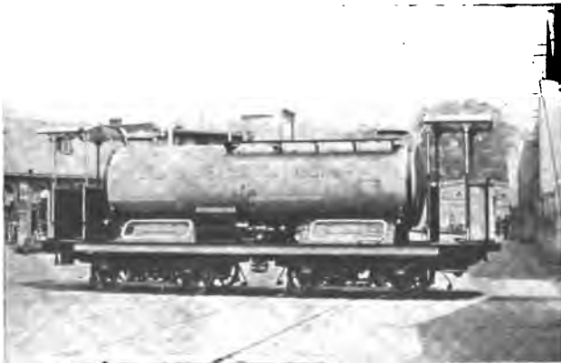
ELECTRIC STREET SPRINKLER USED IN COLOGNE, GERMANY.
