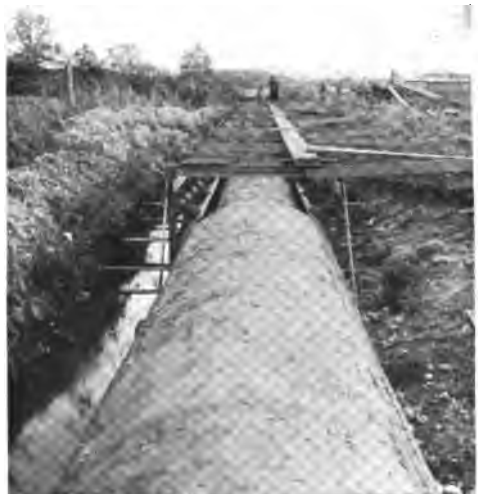
REINFORCED CONCRETE SEWER UNDER CONSTRUCTION AT ST. PAUL, MINNESOTA.
