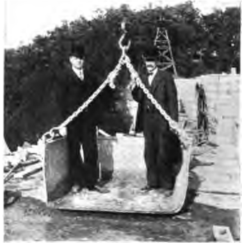
THE MEN WHO PREPARED THE PLANS FOR THE WALNUT LANE BRIDGE.
