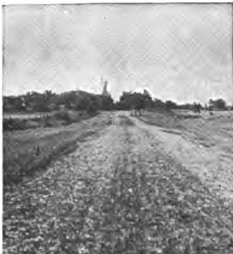
EXPERIMENTAL ROAD NEAR PRINCETON, MINN., BUILT OF SAND AND CLOVER.
