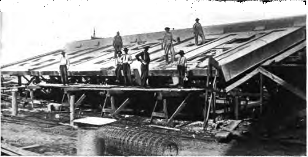
CONSTRUCTING A CONCRETE WALL FOR A HOUSE.
