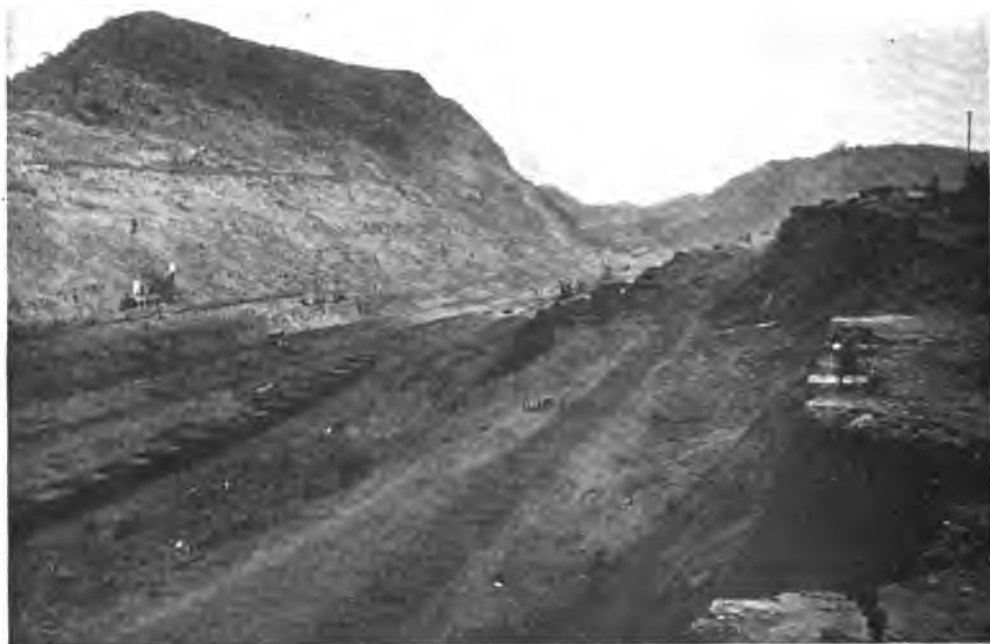
A VIEW OF CULEBRA CUT—LOOKING SOUTH.
