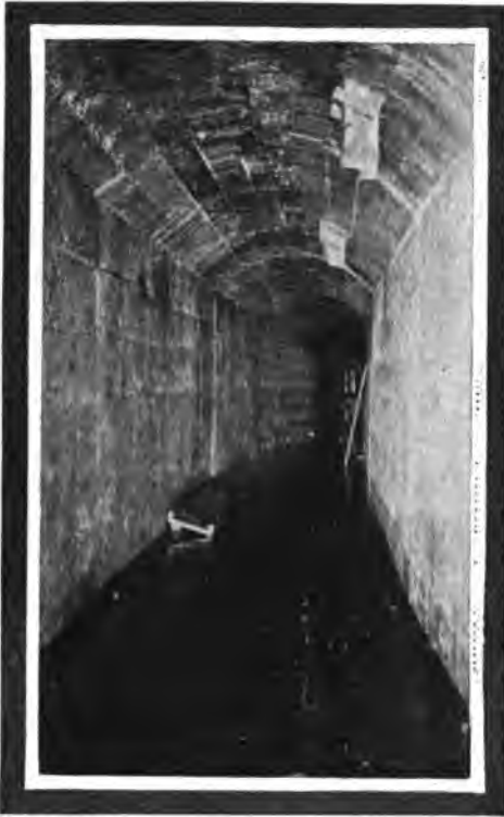
VIEW INSIDE THE COMPLETED TUNNEL.
