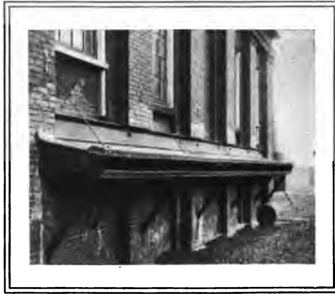
OBSERVATION HOUSE. Miners stand within this protection and watch explosions of coal dust and fire damp in galleries 60 feet away.
