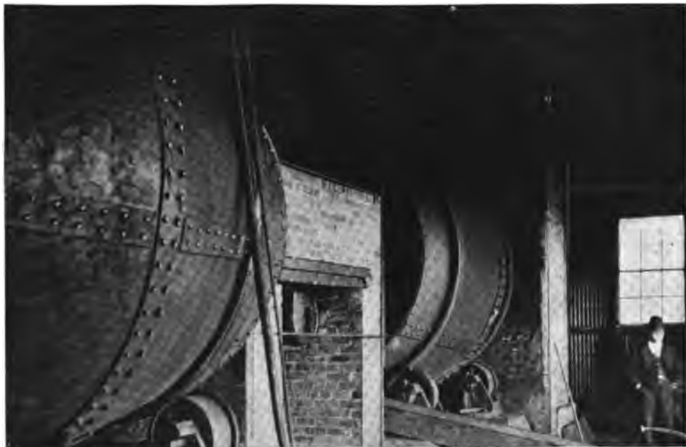
THE ROTARY CYLINDERS AND CONNECTING CHAMBERS AT CLOSE VIEW.
