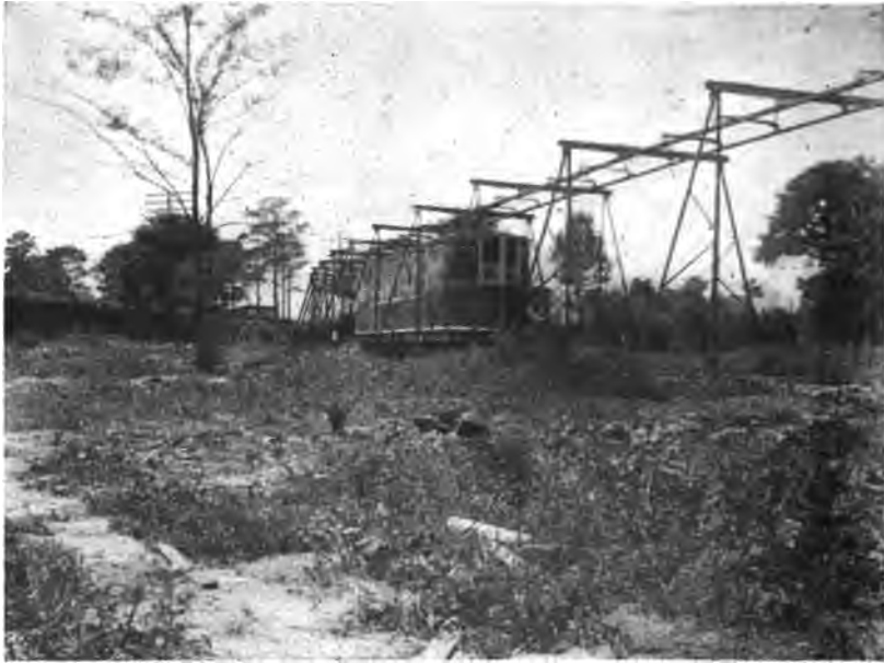
THE MONORAIL HAS POINTED ENDS TO LESSEN AIR RESISTANCE.
