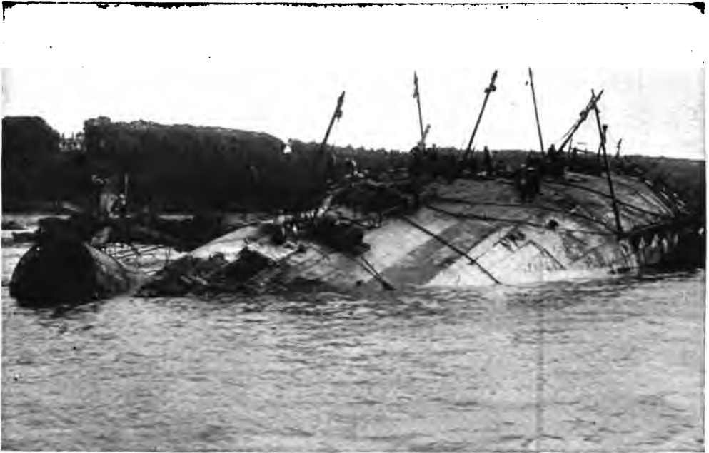
BEGINNING SALVAGE OPERATIONS.
