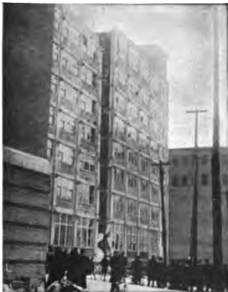
THE BUILDING THROUGH WHICH HUGE TANK FELL.
