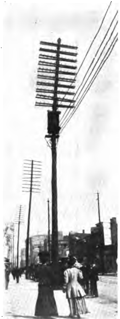
THE OVER-LOADED AND UNSIGHTLY WOODEN POLE.
