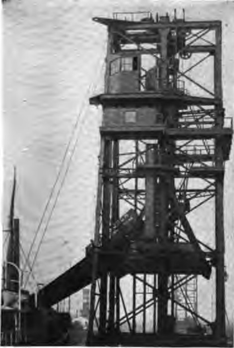
AN HYDRAULIC COAL HOIST IN USE AT LEITH, ENGLAND.
