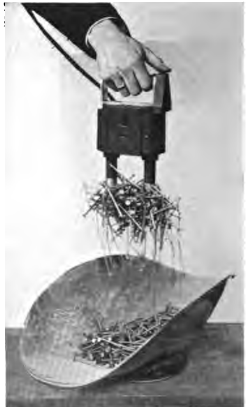
HANDLING NAILS IN BULK BY ELECTRO-MAGNET.
