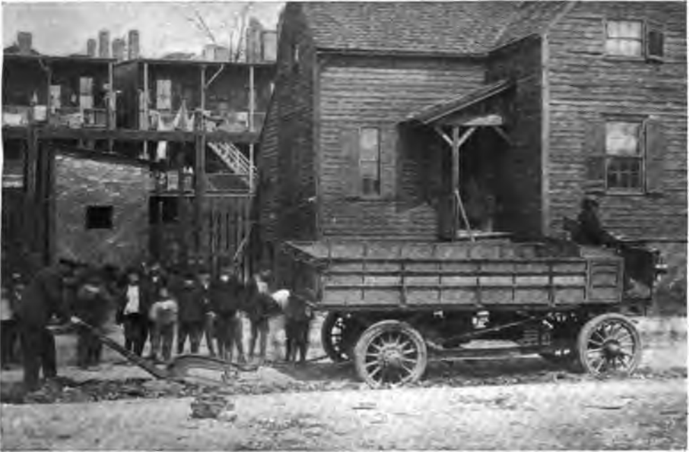
AUTOMOBILE PLOWING TRENCH IN STREET FOR GAS PIPES.
