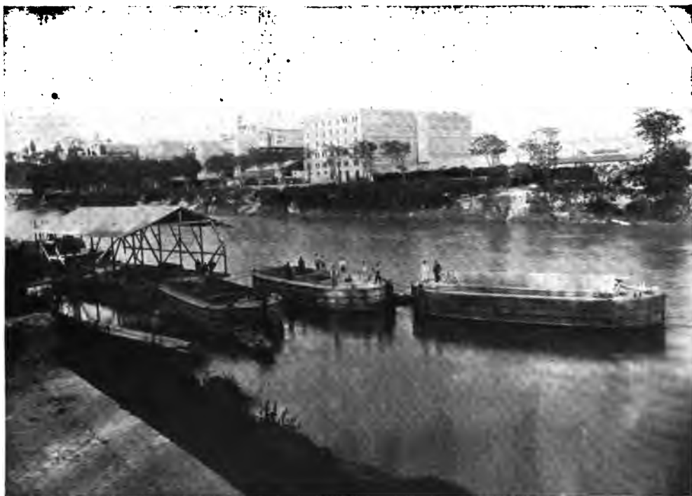
IRON-CONCRETE BOATS BUILT FOR THE ITALIAN NAVY.
