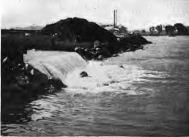
END OF AIR LIFT FLUME, THROUGH WHICH 50,000,000 GALLONS OF WATER PASSED EVERY TWENTY-FOUR HOURS.
