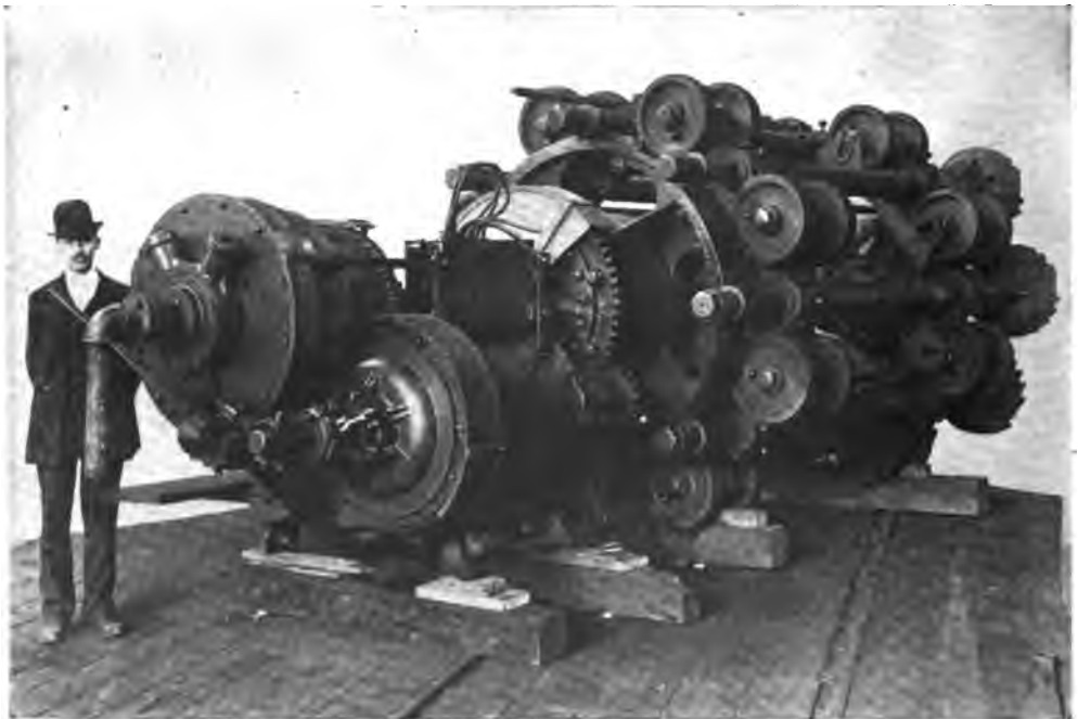
THE TUNNEL DIGGER AS SEEN FROM THE REAR. SHOWING THE MOTOR.
