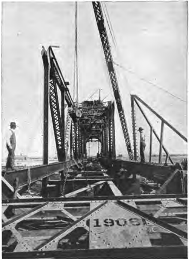
THE HARD-LUCK DRAWBRIDGE UNDER CONSTRUCTION.
