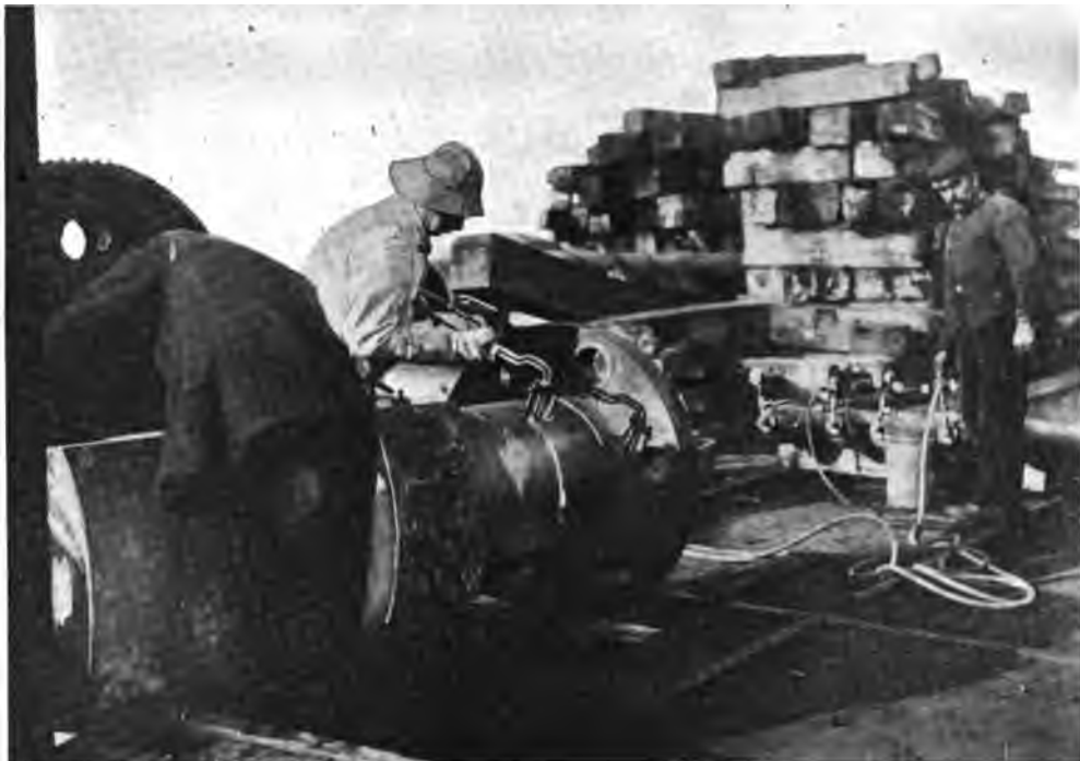
CUTTING A HOLLOW SHAFT OF THREE-INCH THICKNESS.
