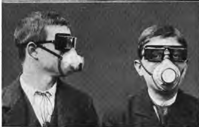
PROTECTION TO EYES AND LUNGS AGAINST DUST AND OTHER FLYING PARTICLES.
