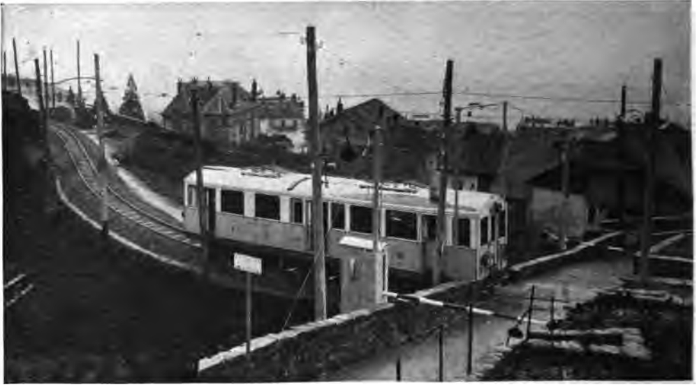
AUTOMATIC ELECTRIC CROSSING GATE NEAR MONTREUX. SWITZERLAND.
