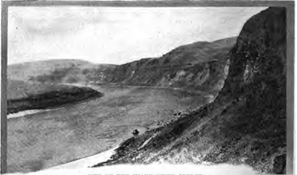
SITE OF THE SNAKE RIVER BRIDGE. One of the streams to be crossed by the North Coast Railway.
