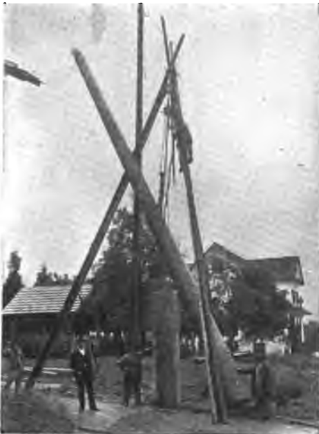
HOW CONCRETE POLES ARE PLACED IN POSITION IN SECTIONS.
