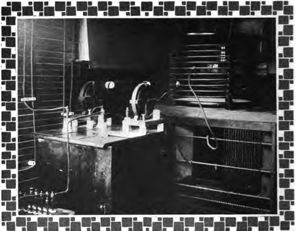
INTERIOR OF HIGH POWER UNITED WIRELESS STATION AT SEATTLE.
