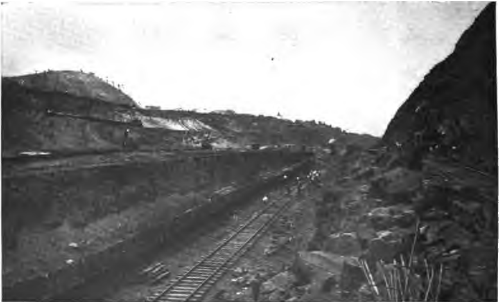
EXCAVATION WORK ON CONTRACTORS' HILL.
