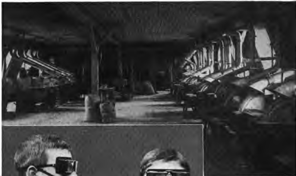
DUST ABSORBING INSTALLATION IN A COMB FACTORY. At every working desk a special aspirator absorbs the obnoxious dust, and draws fresh air into the room.
