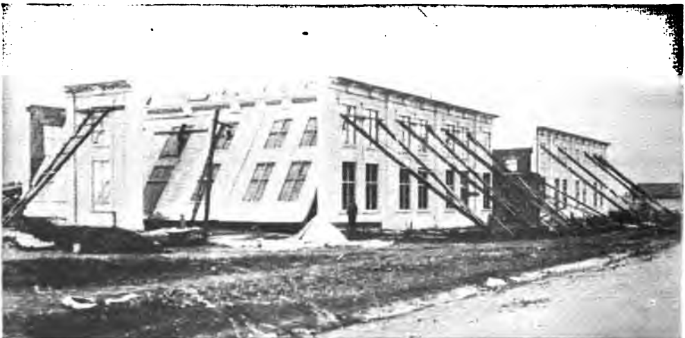
CLOSING UP THE END OF BUILDING CONSTRUCTED OF SEPARATELY MOULDED WALLS.
