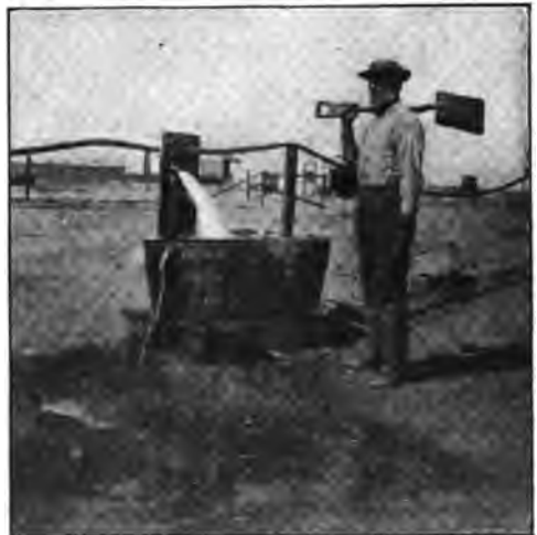
THE WATER EMERGING FROM THE UNDERGROUND RIVER.
