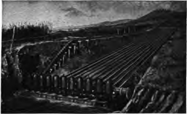
A BATTERY OF HYDRAULIC RAMS FOR IRRIGATING ORCHARD LAND.
