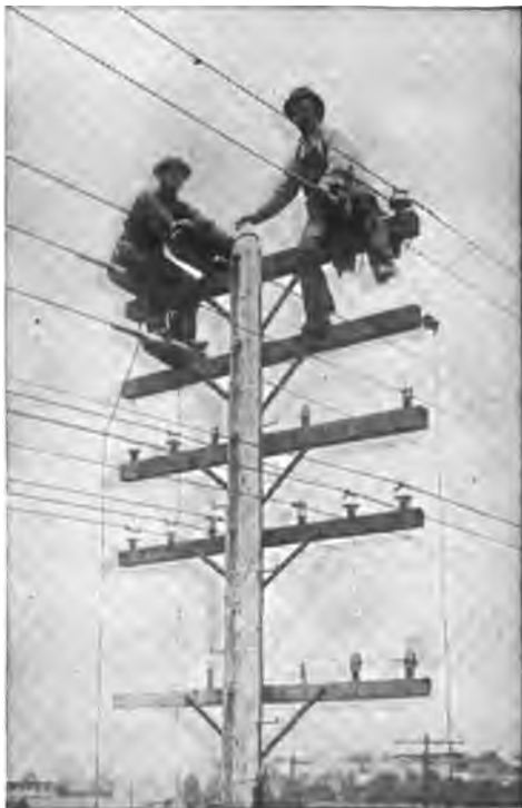
LINEMEN USING SHIELDS AS PROTECTION AGAINST LIVE WIRES.
