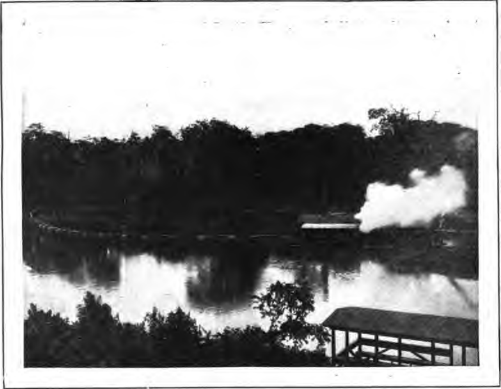
DREDGING THE CHAGRES RIVER. Marsh lands are being drained and reclaimed.
