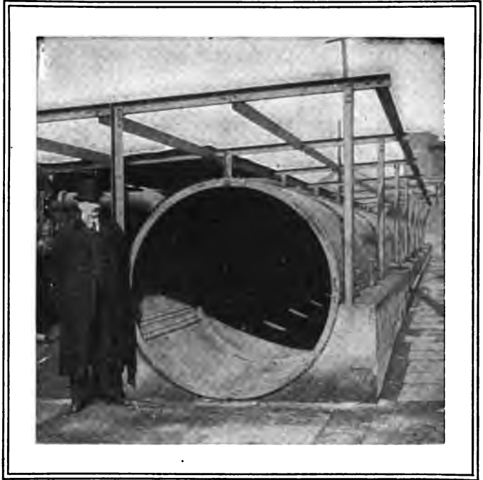
THE EXPLOSIVES CHAMBER, WHERE EXPLOSIVES ARE TESTED IN PRESENCE OF COAL DUST AND FIRE DAMP.
