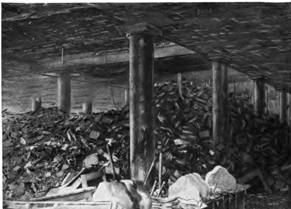
THE PARKER BUILDING FIRE, NEW YORK CITY, JANUARY 10, 1908. Four thousand dollars "saved" on construction, in fireproofing, and $2,000,000 of property destroyed by this false economy.
