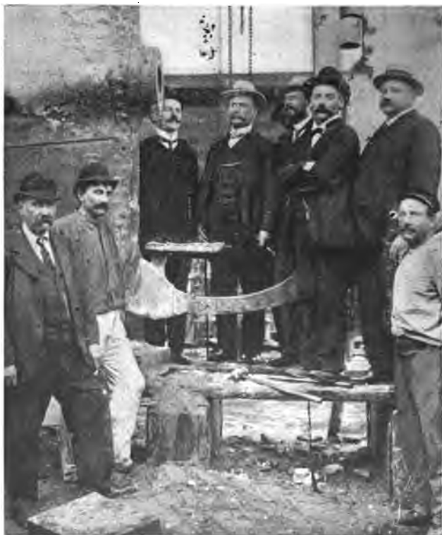
REPAIRING THE STERN-POST OF AN OCEAN-GOING STEAMSHIP.
