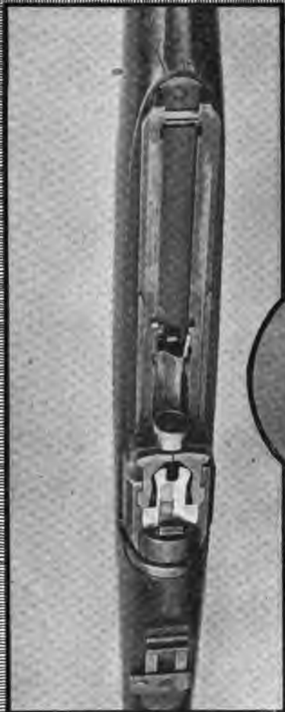
TOP VIEW OF MECHANISM WITH BREECH BLOCK COVER REMOVED.
