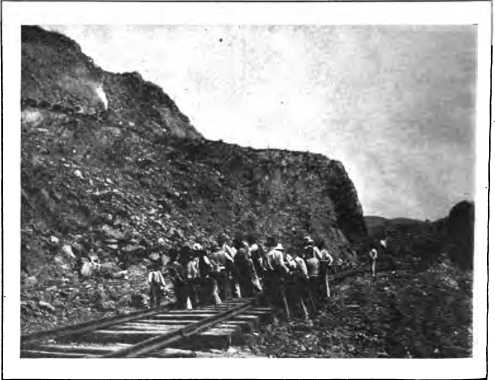
TRACK-SHIFTING BY HAND IN THE BAS OBISPO CUT.
