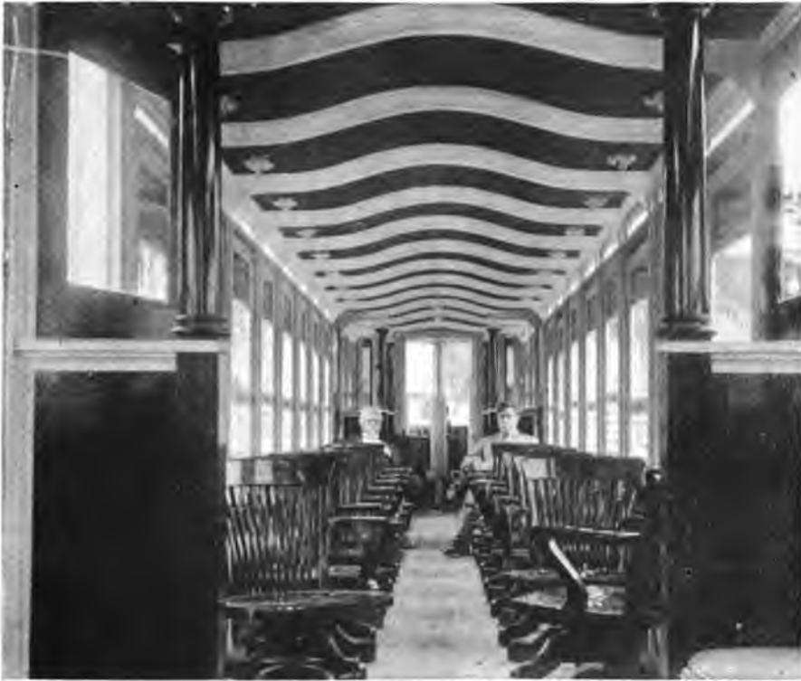
INTERIOR OF THE AMERICAN MONORAIL CAR.
