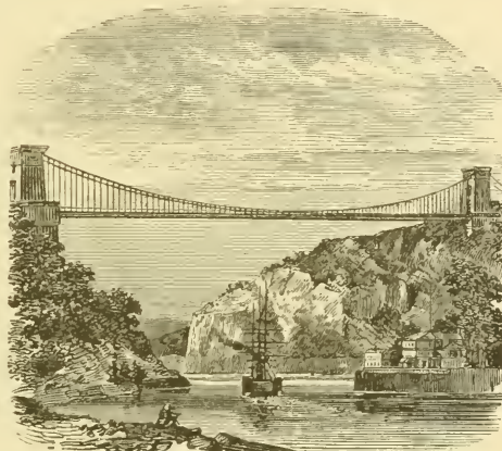
Fig. 66.—CLIFTON SUSPENSION BRIDGE.
