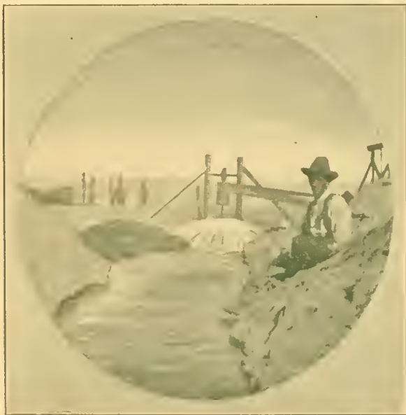
PUMPING PLANT AT DELANO
