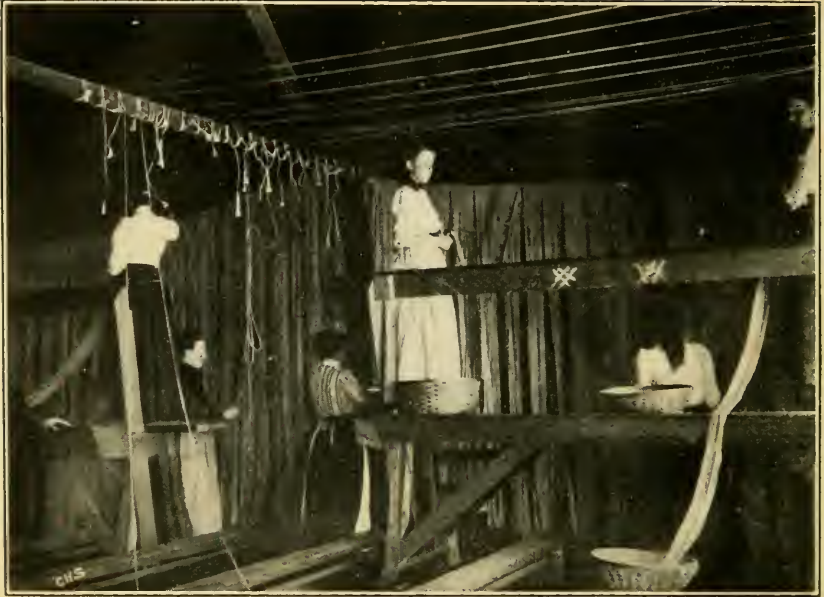
FIG. 1.—DRYING-ROOM OF ISINGLASS FACTORY.
